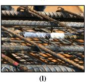
**Figure 3.14. Strain Gauge Installation:**
