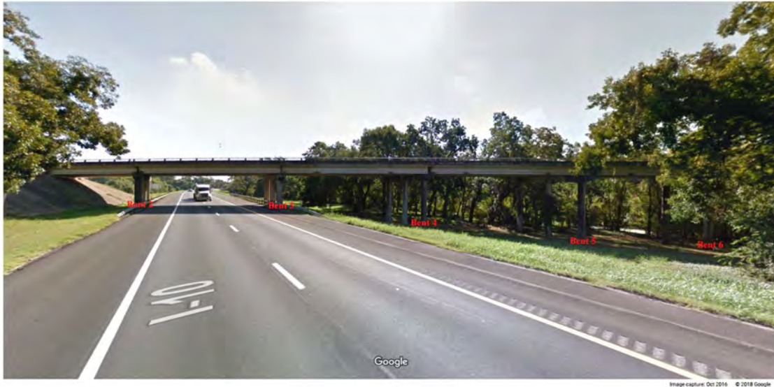
(b) Existing old skewed bridge
