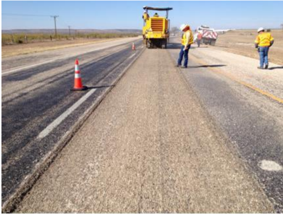
Figure 21. Photos taken from US 87 test site after the milling
