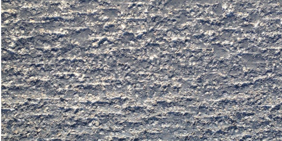
Figure 41. Photo taken from US 277 test site 6 months after the milling
