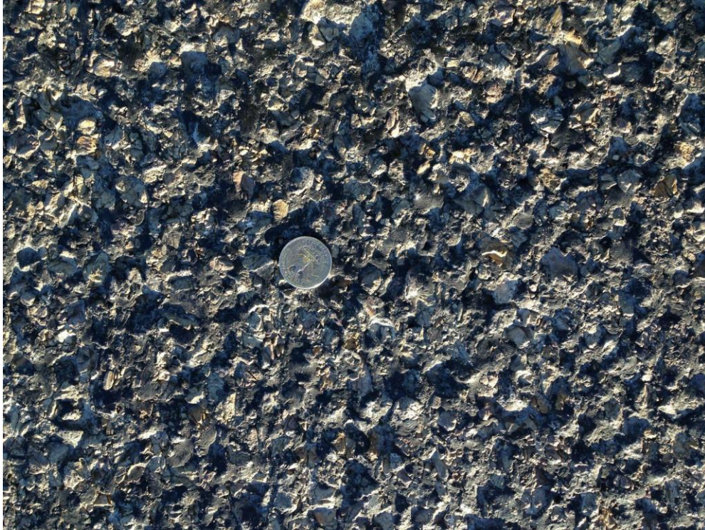
Figure 22. Photo taken from US 87 test site 3 months after the milling
