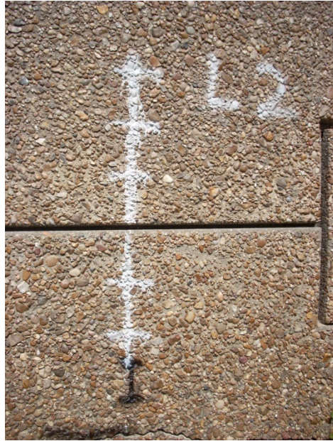
Fig. 5.26. View of L2 Rotation Monitoring Mark Line on the Retaining Wall.
