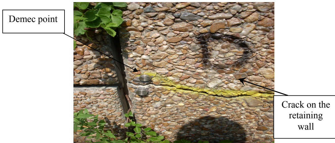
Fig. 5.6. Demec on the Embankment Retaining Wall (Project 3).
