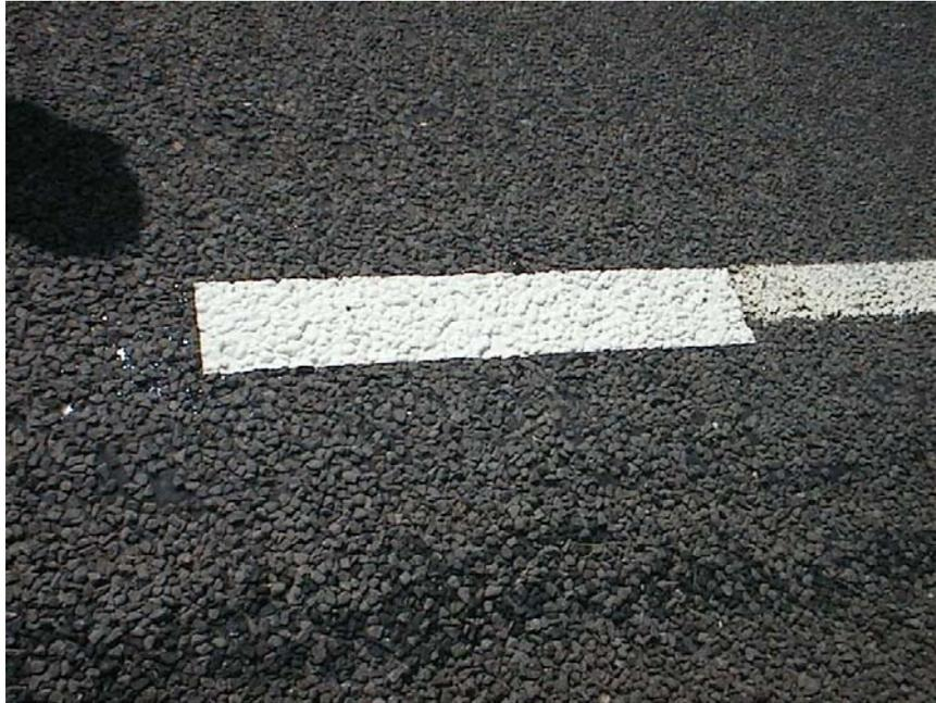
Figure 5.8 (b) TPMM on new pavement with rough surface in Waco District
