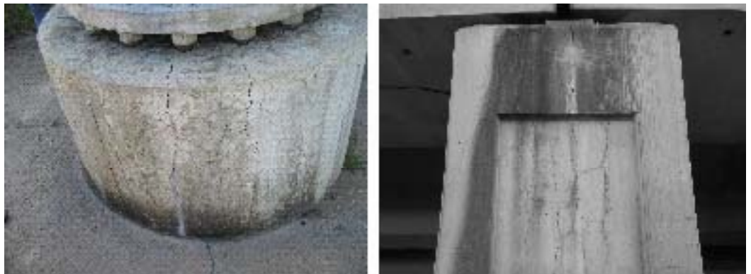
Figure 1 – Examples of structures affected by ASR and/or DEF in the state of Texas
