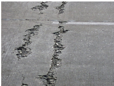
Figure 1 – Severe Spalling of CRCP (Won, 2001)
