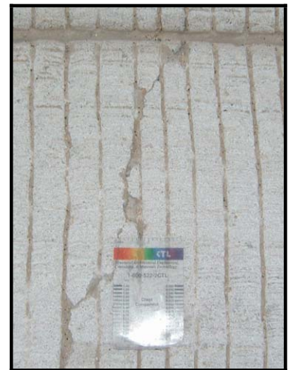
Figure 5 – Evidence of Spalling in Control Sections after 235 days (note that no spalling has been observed in any of the FRC sections)
