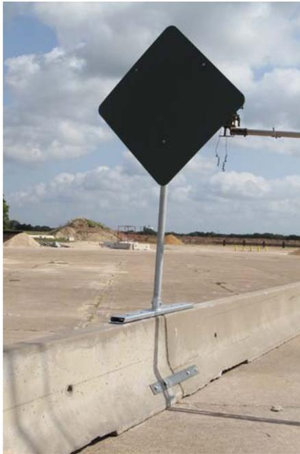
**Figure 1: Sign Support Assembly Anchored to the Top of the TxDOT Type 2 PCTB.**
