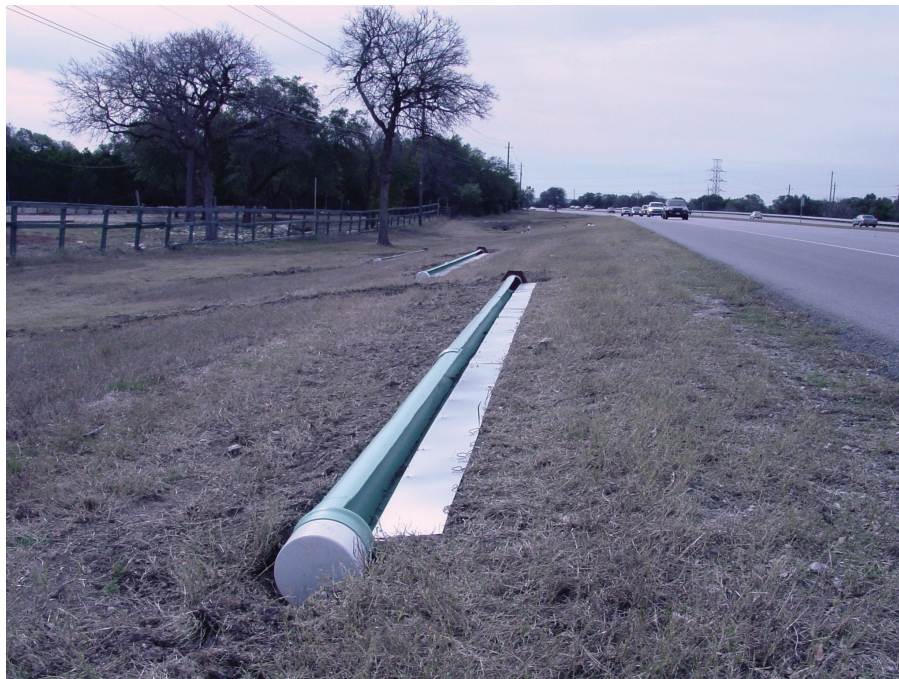
Figure 1: Photograph of installed collection pipe at Austin Site 2
