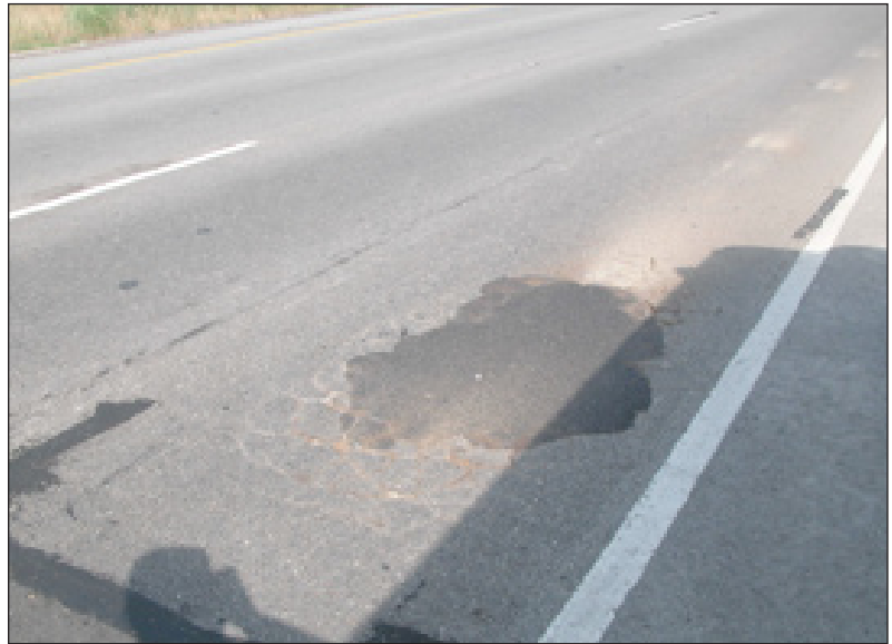
Figure 1. Premature Failure of a Pavement Attributed to Moisture-Susceptible Base.
