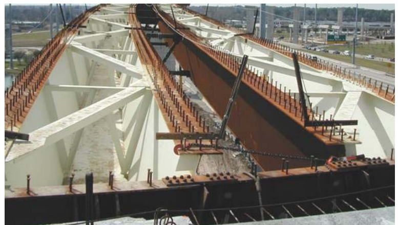
Figure 1 Box girder bracing systems
