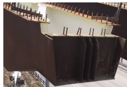
Figure 2 Partial depth end diaphragm (soft end panel)
