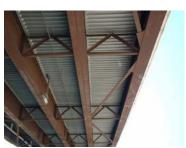
Figure 1 Cross-frames used to reduce unbraced length of girders
