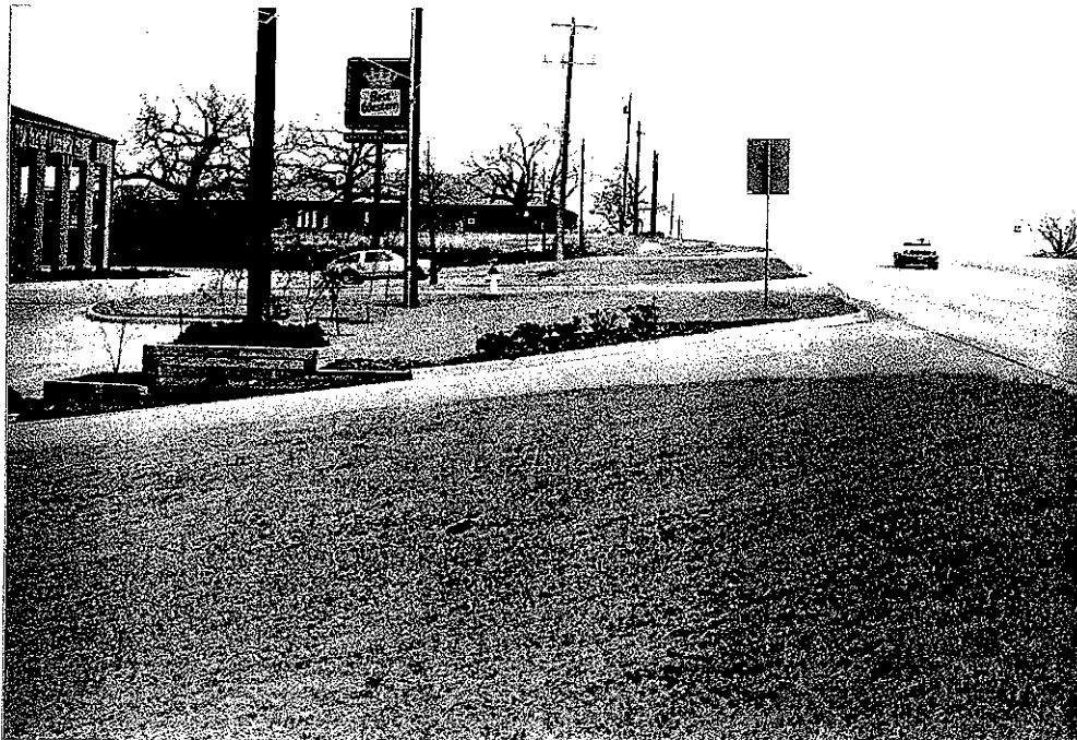
Figure A-5. The first grade descending from the minor arterial is of adequate length, but the slope may be inappropriate for high volume commercial operations. ( G_1 = -4\% , L_1 = 50 ft.)
