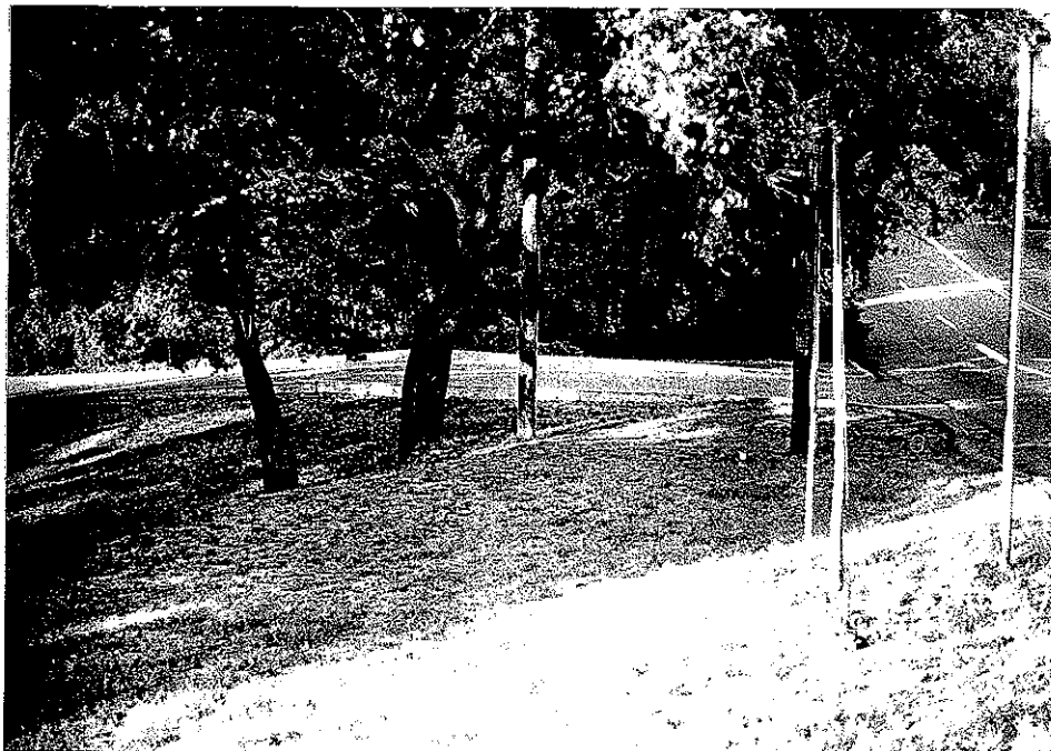
Figure A-6. Long grades and relatively minor changes in grades are characteristics of good design. The dimensions for this driveway are acceptable for commercial operations with low to moderate volumes. Unfortunately, the trees may interfere with adequate sight distance. ( G_1 = 1.5\% , L_1 = 45 ft., G_2 = -3\% , L_2 = 45 ft.)
