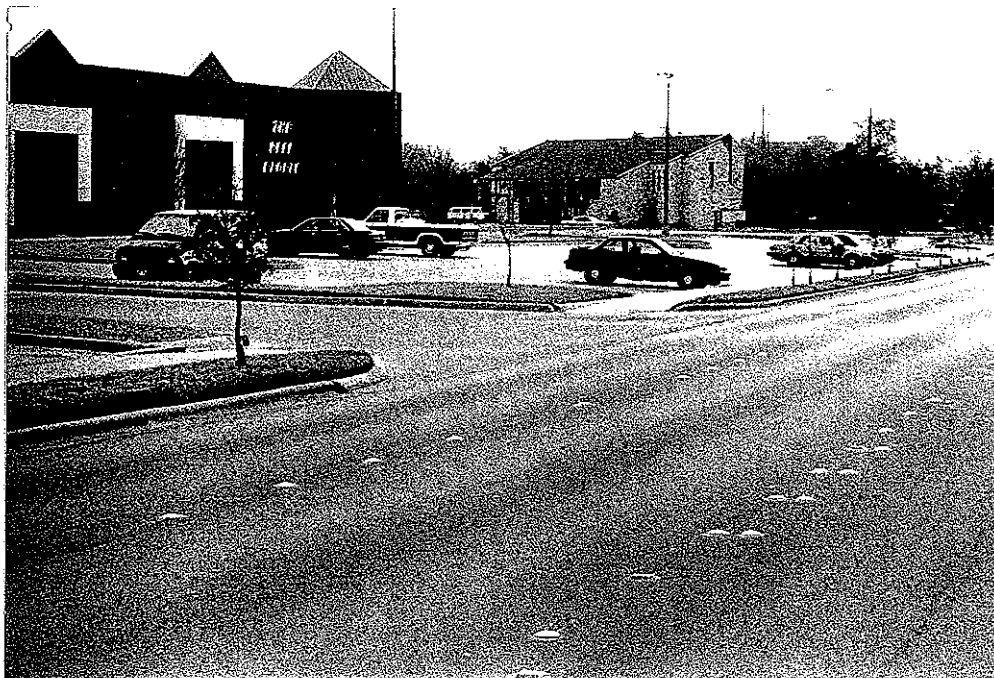
Figure A-8. A smooth grade with a high point 6 inches above the flow line of the gutter, at a distance of about 25 feet from the curb line, provides a good design for a commercial driveway on a major urban street. The profile results in a comfortable ride for occupants and sufficient control of water flowing in the gutter section. ( G_1 = 2\% , L_1 = 25 ft., G_2 = -1.5\% , L_2 = 45 ft.)
