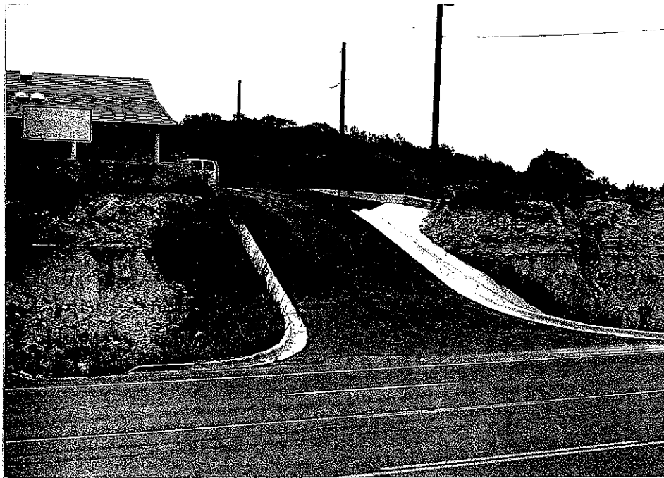
Figure A-1. The widening of a rural highway has produced a driveway with a severe grade. Driver attention is focused on the driveway rather than the highway, and multiple hazards are presented for entering and exiting vehicles. Deep scrape marks exist in the pavement from impacts with vehicle bumpers and under-carriages. ( G_1=2\% , L_1=34 ft., G_2=22\% , L_2=65 ft.)
