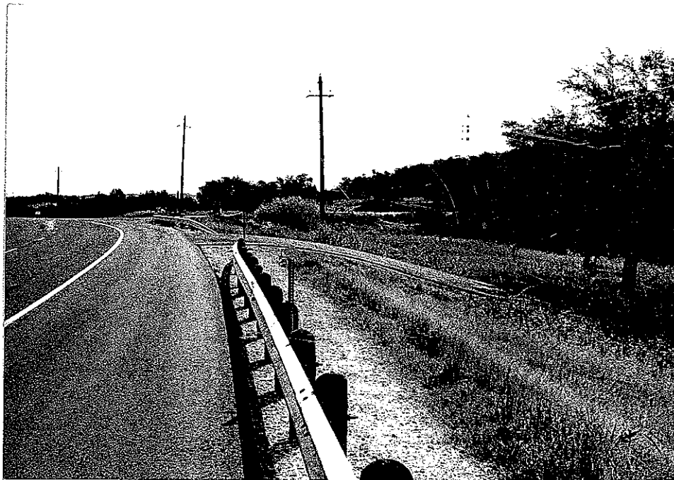
Figure A-4. The initial grade of this driveway may be too short to accommodate a high volume of large trucks; note, however, that the first grade corresponds to the shoulder's slope and continues for several feet beyond the shoulder's edge. The driveway's second grade is severe and may limit the sight distance of drivers attempting to exit from the property. ( G_1=4.5\% , L_1=20 ft., G_2=-16\% , L_2=50 ft.)
