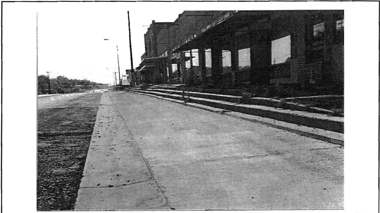
Figure C-1 Reduced Parking from Head-In Angle to Parallel Parking in Front of Old Businesses in Old Building
