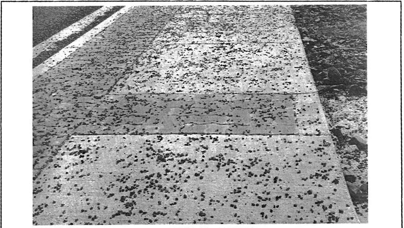
Figure C-8 New Ornamental Sidewalks Built on Each Side of the Widened Facility
