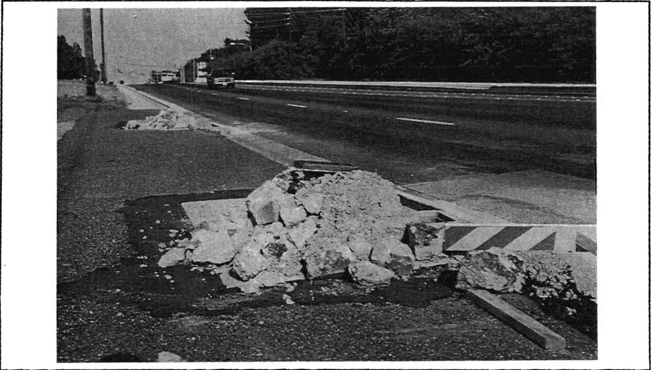
Figure C-7 Reworking Storm Sewer Openings at Previously Widened Intersections
