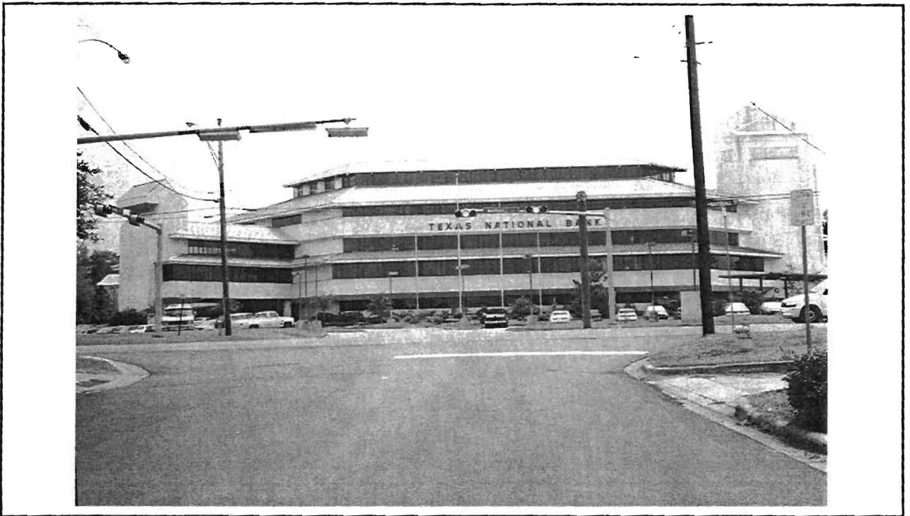
Figure C-11 Finished Facility in Front of One of the Existing Businesses
