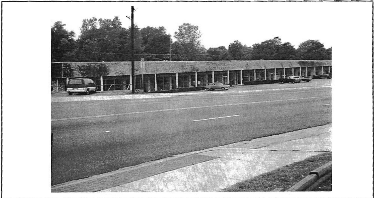
Figure C-10 Finished Facility Showing Curbing, Driveways, Sidewalks, and Continuous Two-Way Left-Turn Lane
