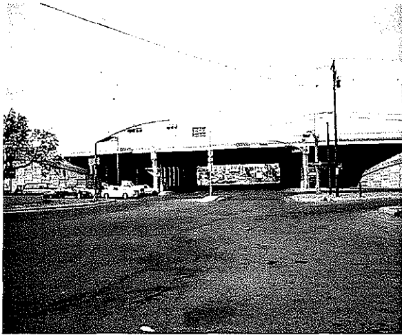
FIGURE 34. EXISTING OVERPASS AT AIRWAY & I-10.
