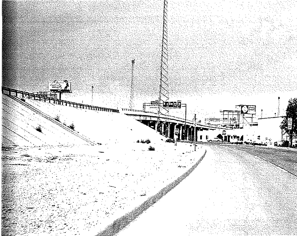
FIGURE 9. TYPICAL RIPRAP SLOPES AS SEEN FROM FRONTAGE ROAD.
