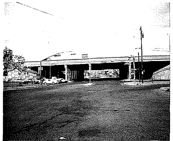
FIGURE 37. ACCENT COLOR EXTENDED TO RETAINING WALL.
