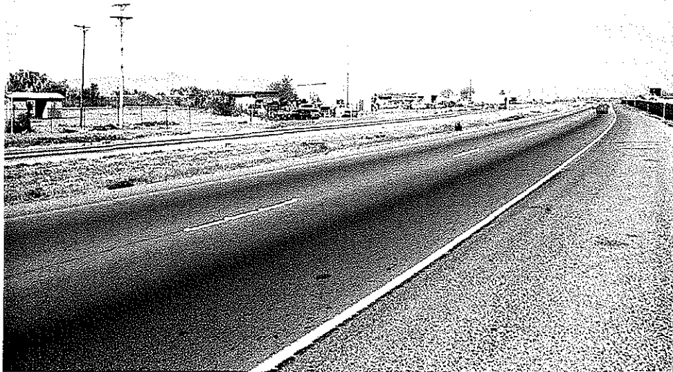
FIGURE 21. UNSCREENED COMMERCIAL AREA ON BORDER HIGHWAY.
