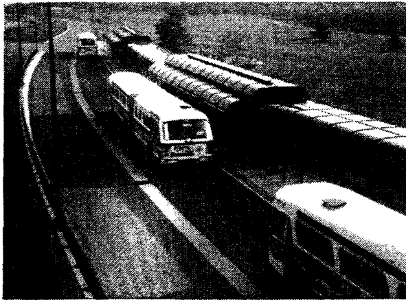
Exclusive HOV Facility on Separate Right-of-Way, Ottawa Transitway, Canada
