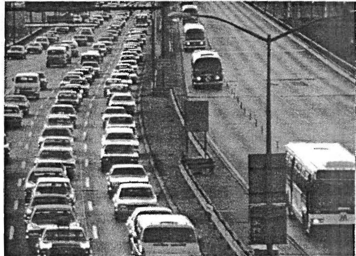
Contraflow Lane, Gowanus Expressway, New York City
