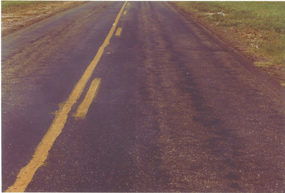
Figure 13. Category B Surface
