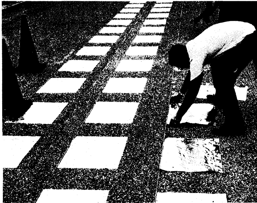
Figure 5. Application of aluminum foil envelopes to the roadway.
