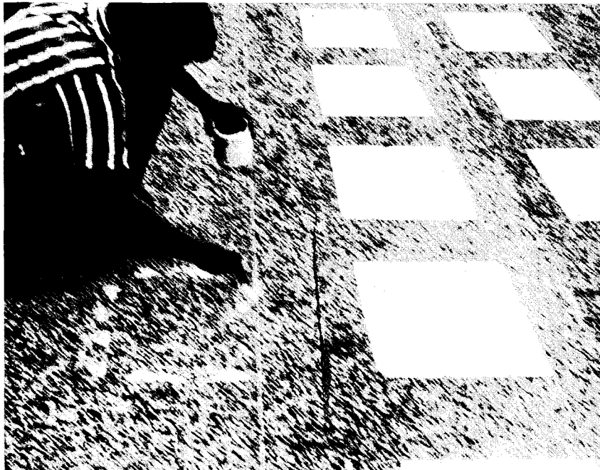
Figure 4. Application of contact cement to the roadway.
