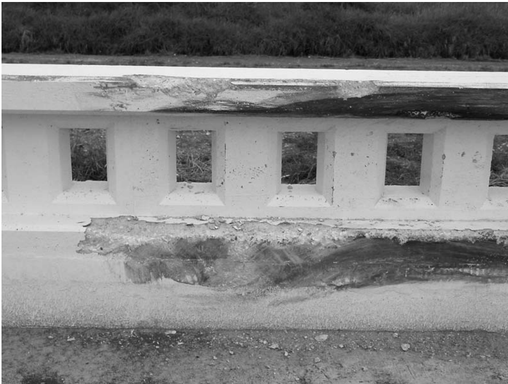
Figure 6. Installation after Test No. 421324-3.
