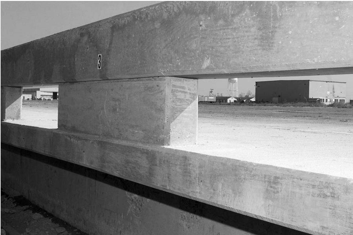
Figure 15. Texas T202 (MOD) Bridge Rail with GFRP.
