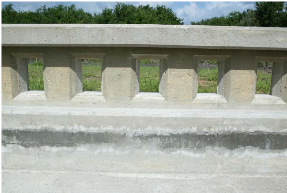
Figure 10. Texas Type F411 Bridge Rail.
