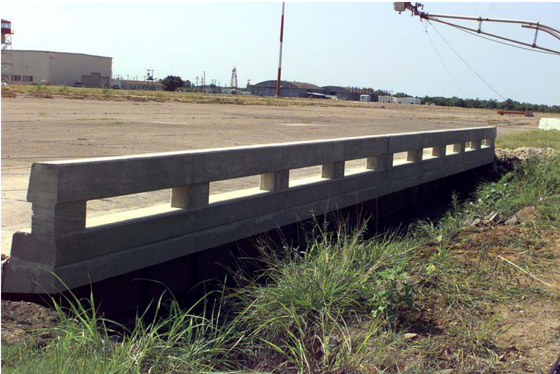
Figure 8. Natchez Trace Bridge Rail.
