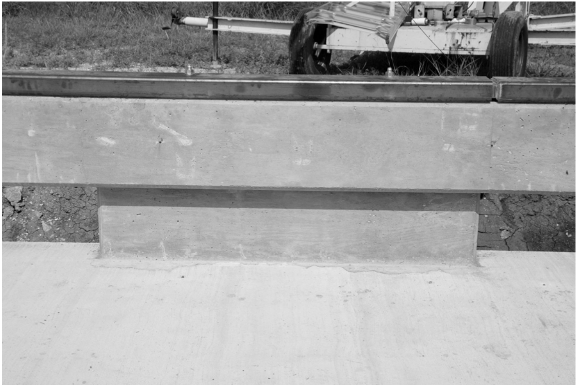
Figure 17. Texas T202 (MOD) Bridge Rail with GFRP and Metal Rail.
