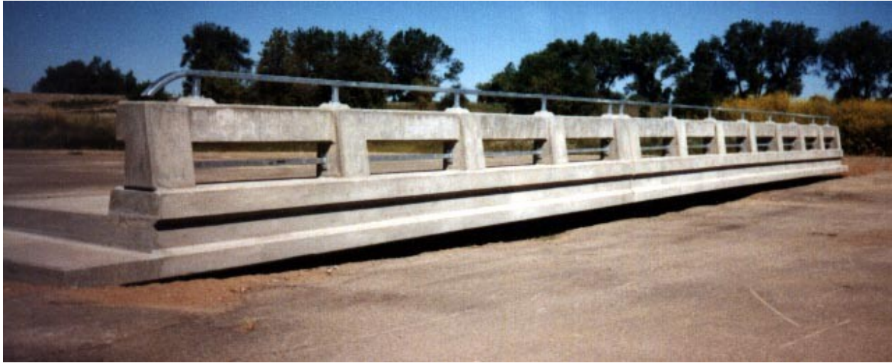
Figure 12. Type 80SW Bridge Rail with Sidewalk.
