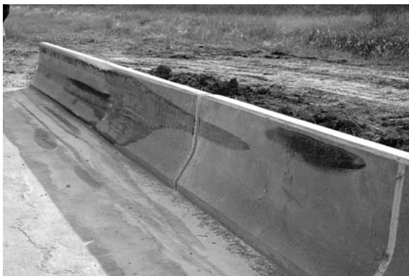
Figure 7. Installation after Test 421323-1.
