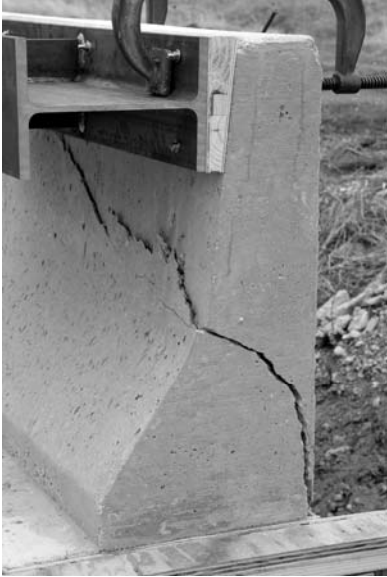
Figure 20. Failure Mode for Test 421323-S1.
