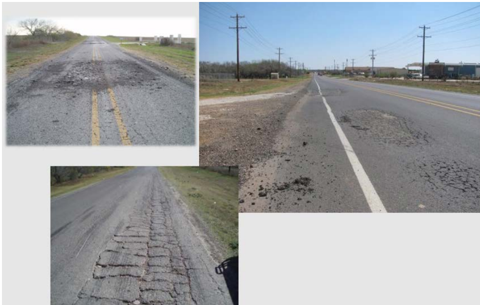
Figure 26. Roadway Damage Due to Heavy Trucks.
