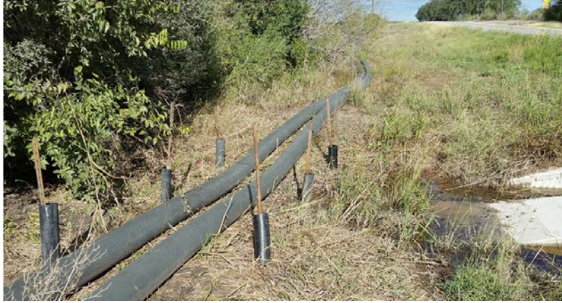
Figure 39. Example of Temporary Waterline in State Roadway Right of Way in Texas.
