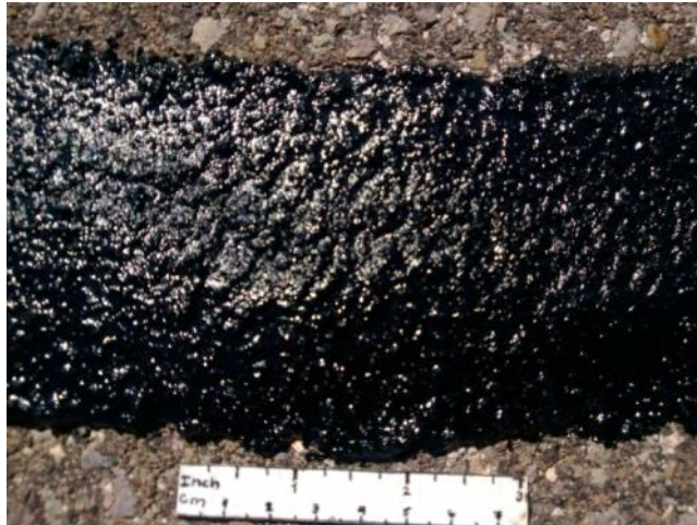
(b) New Pavement, Route
