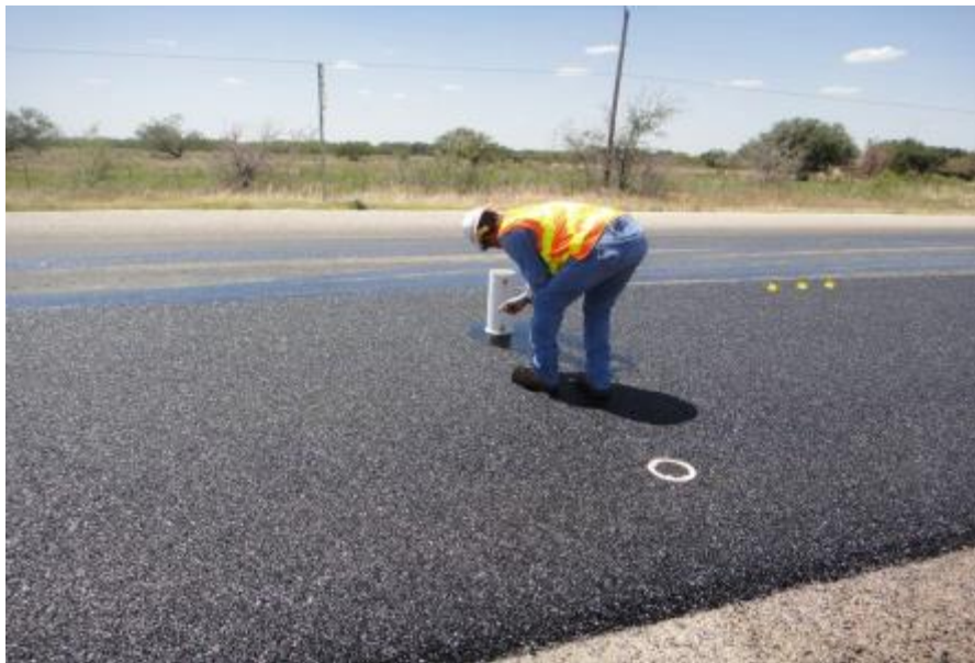
Figure 22. Water Flow Testing on US 183 Fine PFC.
