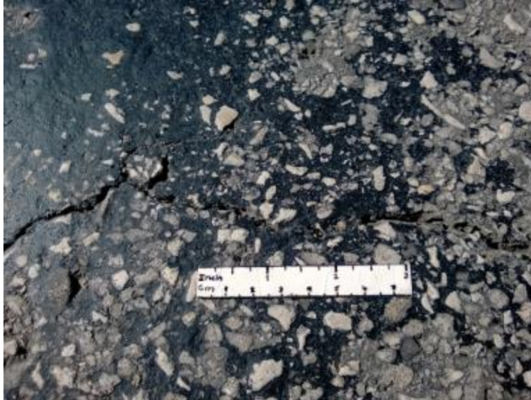
Figure 30. Existing Crack.
