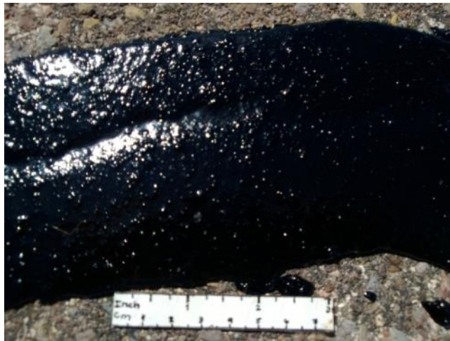
(b) New Pavement, Route
