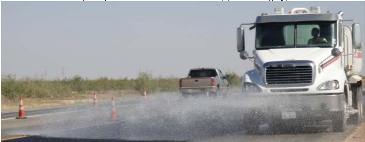
c) Sprinkling before opening the PFC to traffic
