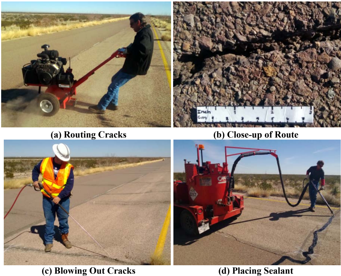
Figure 7. Crack Sealant Construction.
