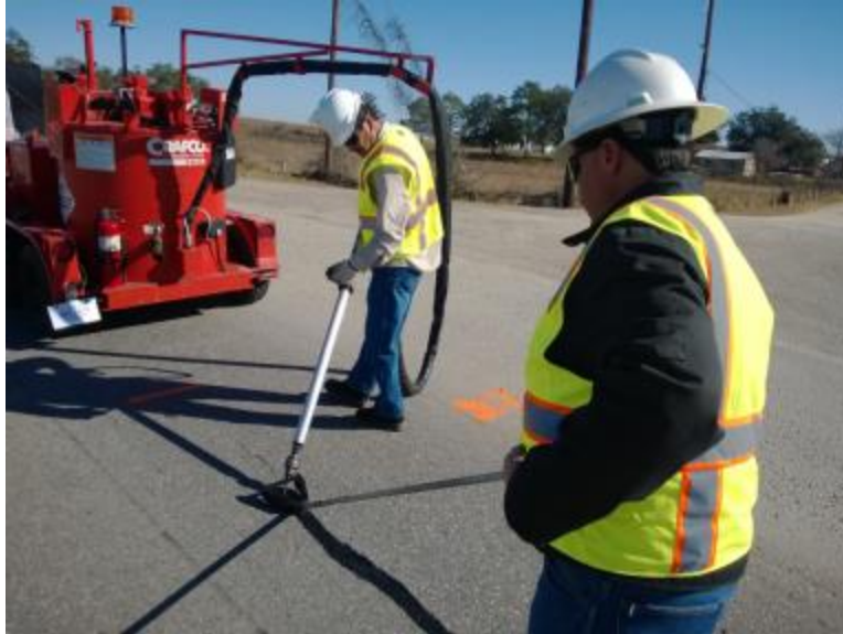
Figure 32. Crack Sealant Construction.
