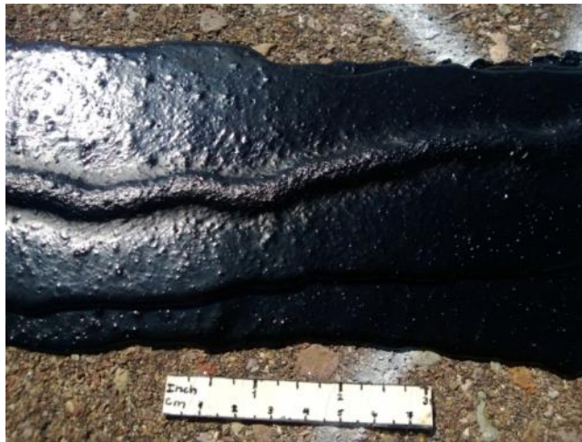
(b) New Pavement, Route
