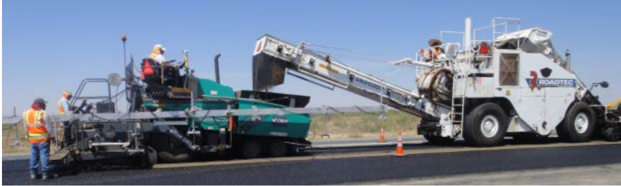
a) Belly dump trucks with RoadTec pick up
