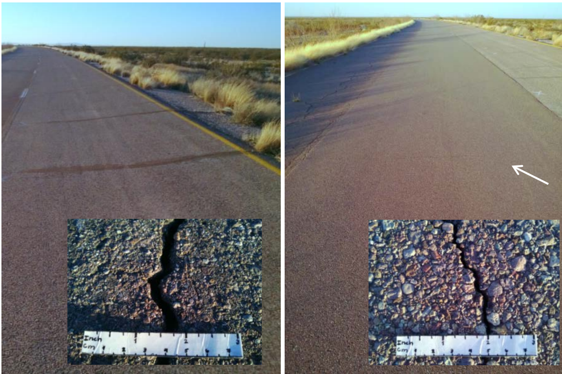
(a) Outer Lane (Older Pavement)
