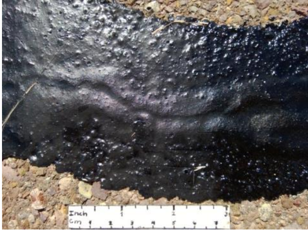
(a) New Pavement, No Route
