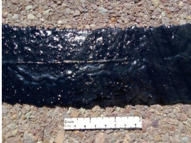
(a) New Pavement, No Route
