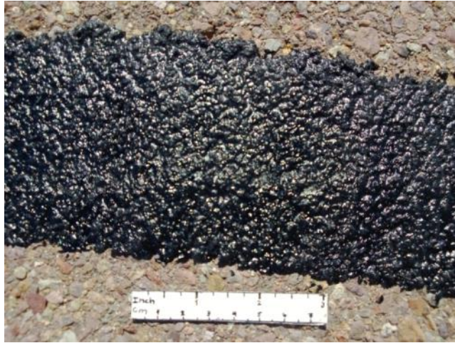
(a) New Pavement, No Route
