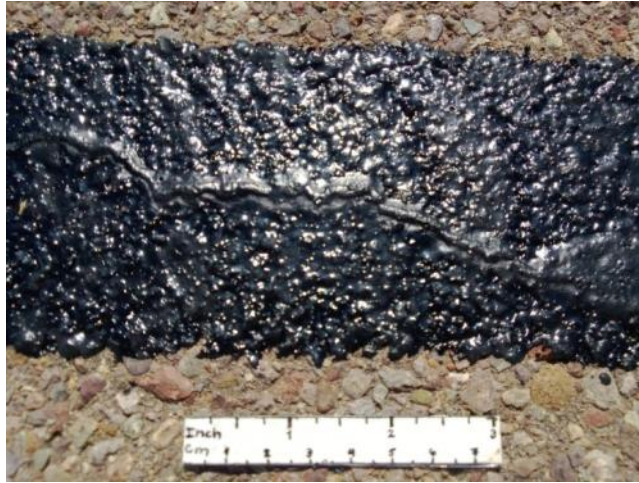
(a) New Pavement, No Route
