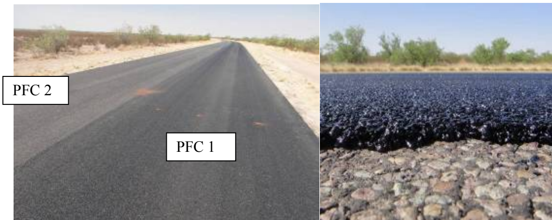
Figure 17. PFC Mix on Pecos Facility Entrance Road.
