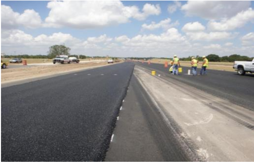
Figure 20. Construction of the Bryan Fine PFC Exit Ramp.
