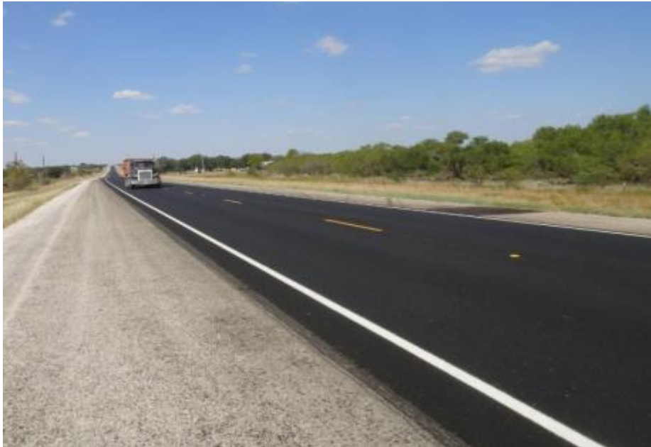
Figure 23. US 183 PFC Three Months after Construction.
