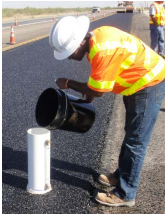
Figure 26. Water Flow Being Conducted on the New PFC.
