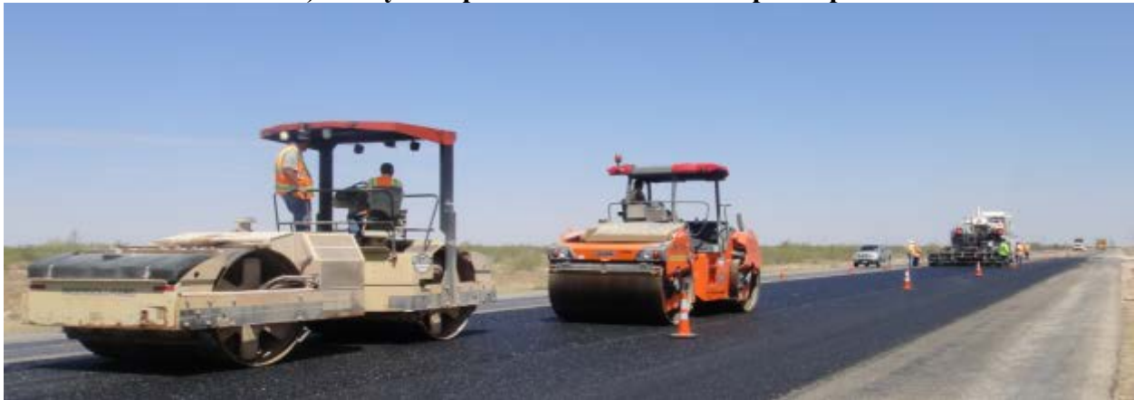
b) one pass of two steel wheel rollers, (no backing up)
