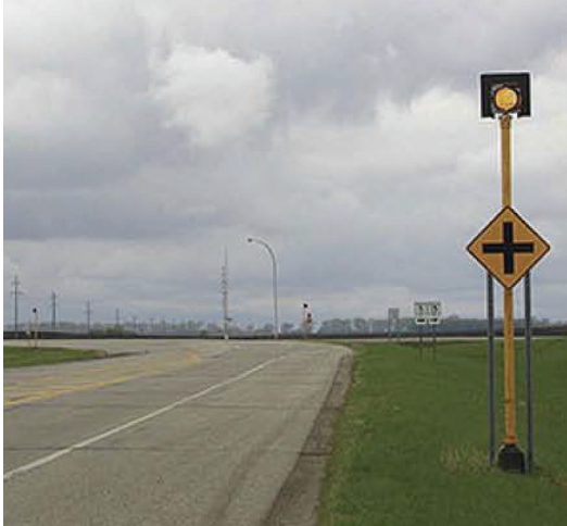
Figure 8. Examples of Replacement Beacons for Overhead Flashing Beacons.
