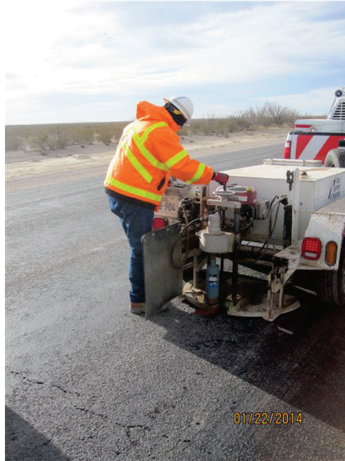
Figure 24. Core Machine Preparing the Pavement to Install the Sensors.
