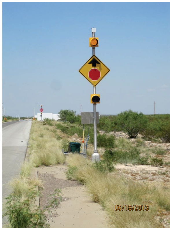
Figure 20. Stop Ahead Sign Installed at Pecos Test Track.
