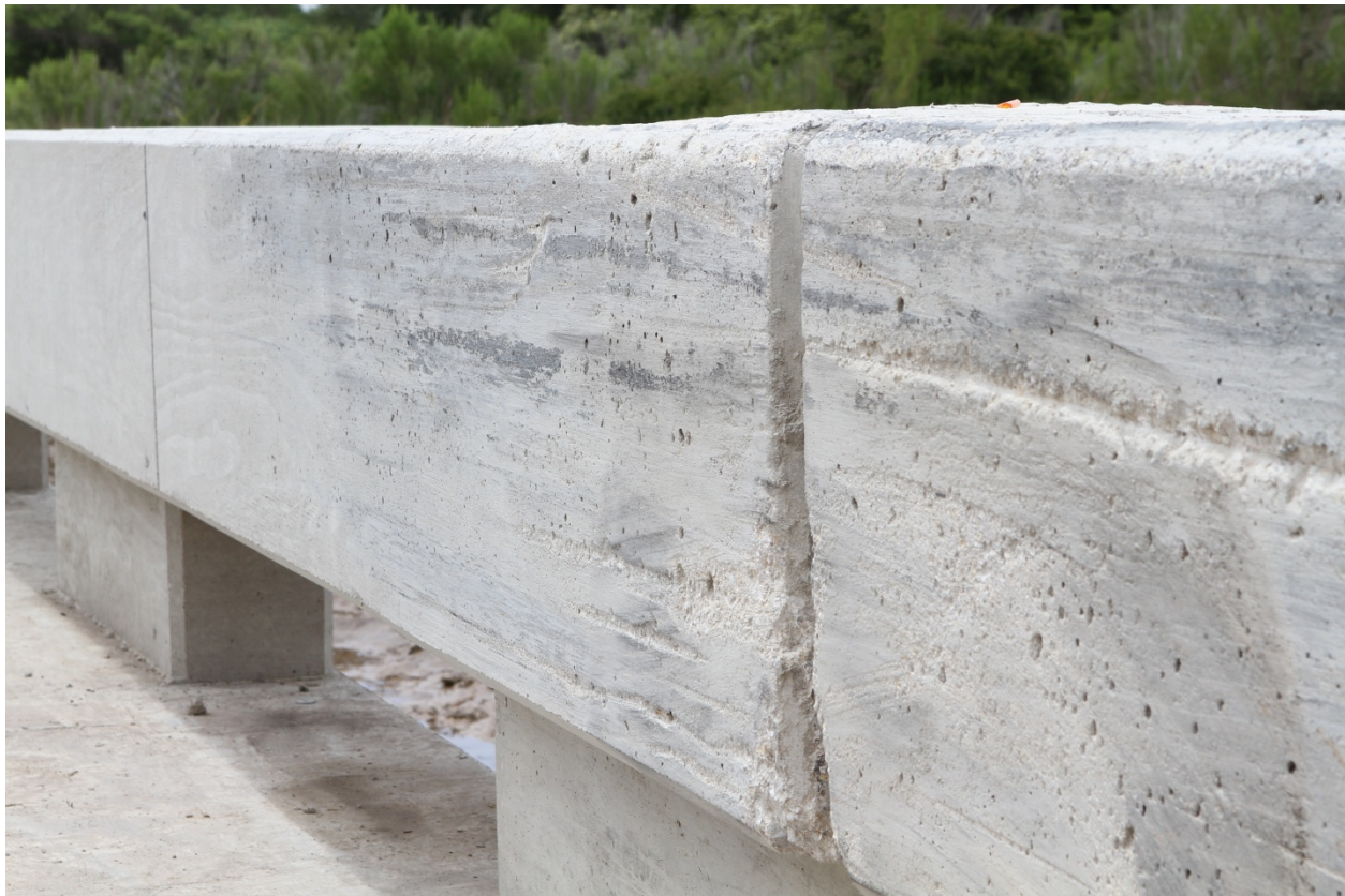
Figure 7.4. Installation after Test No. 420021-5.
