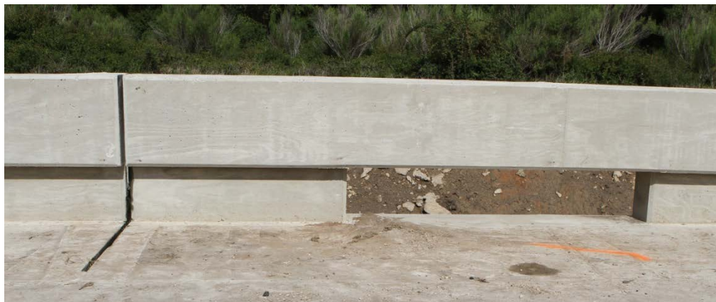
Figure 4.4. 5-inch CIPD Barrier Anchor Installation before Test No. 420021-5.
