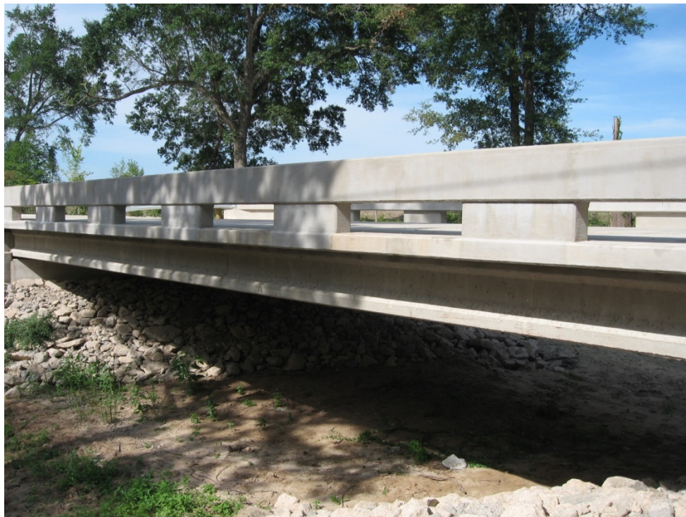
Figure 2.1. TxDOT T223 Barrier.
