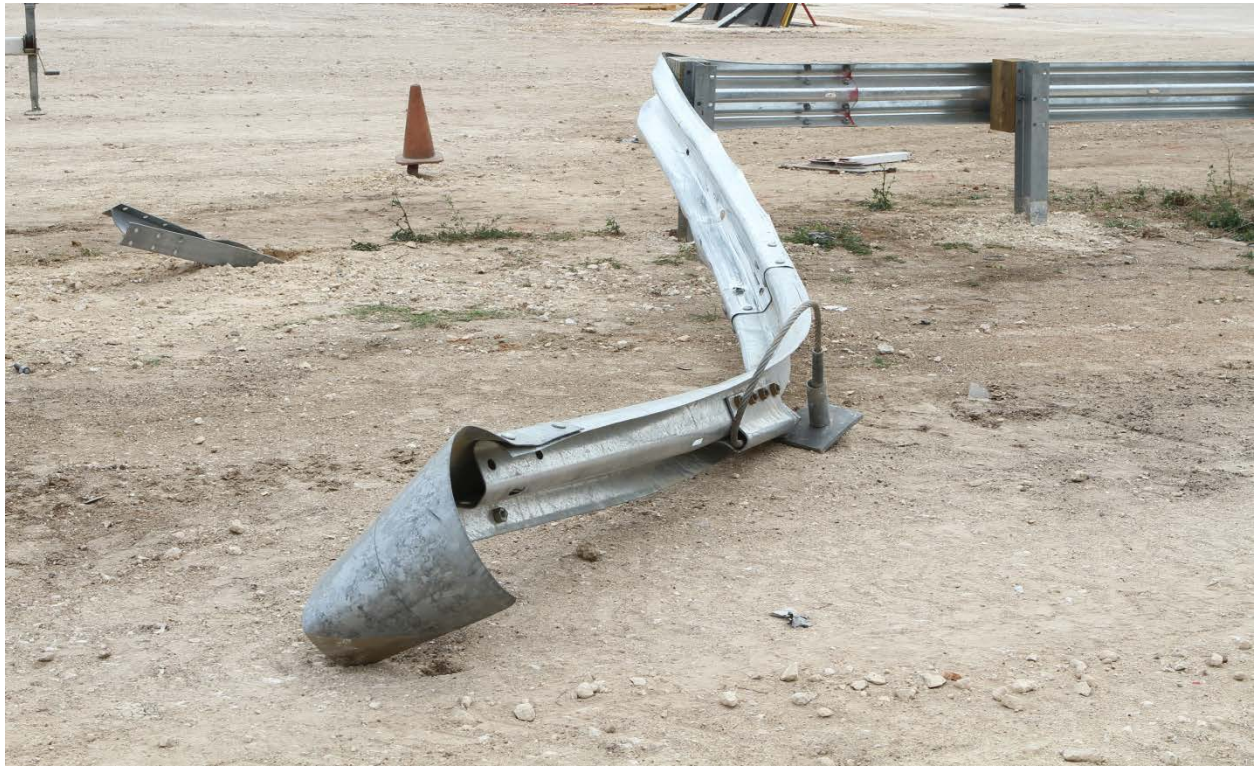
Figure 5.4. Installation after Test No. 420021-1.
