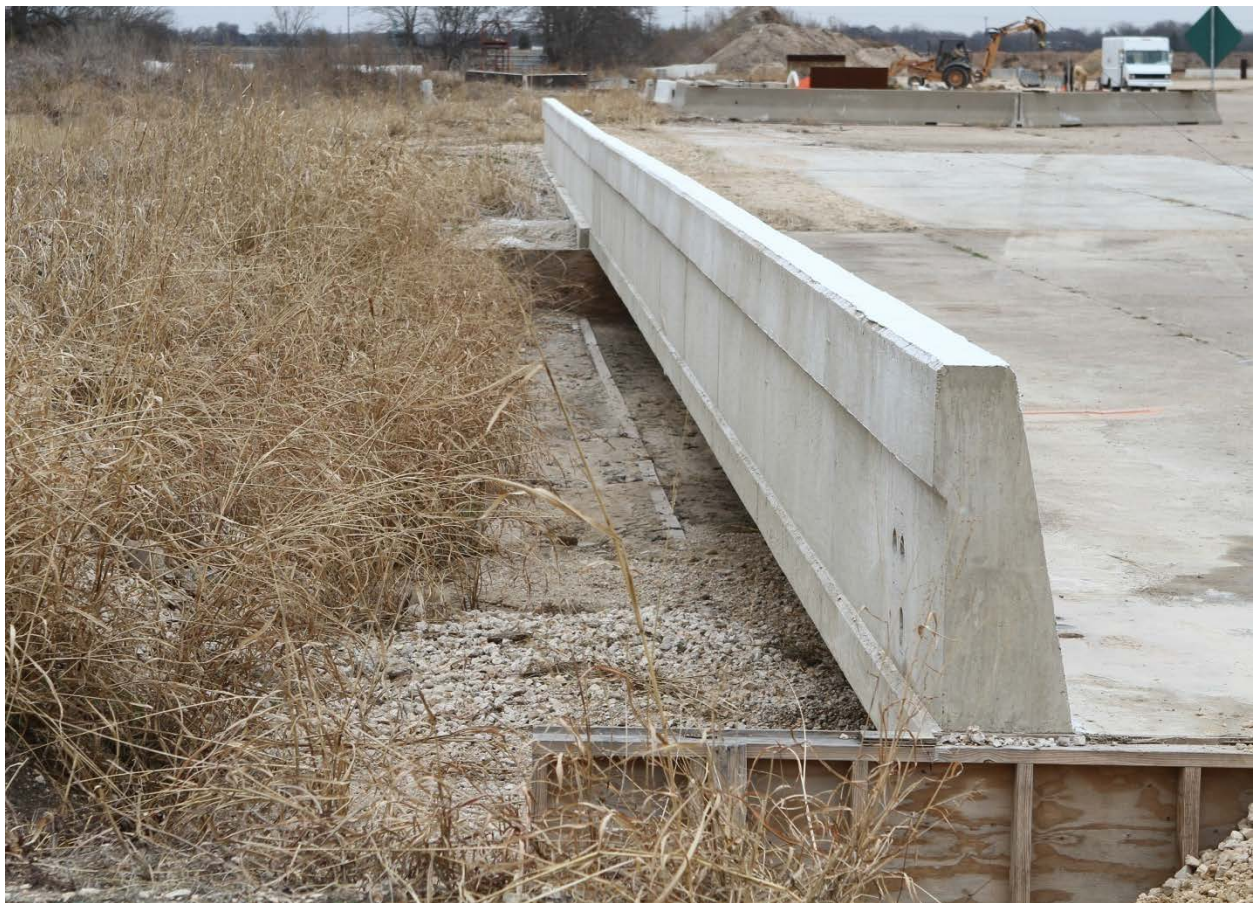
Figure 3.4. TxDOT Single Slope Traffic Railing (SSTR) before Test No. 420020-9b.
