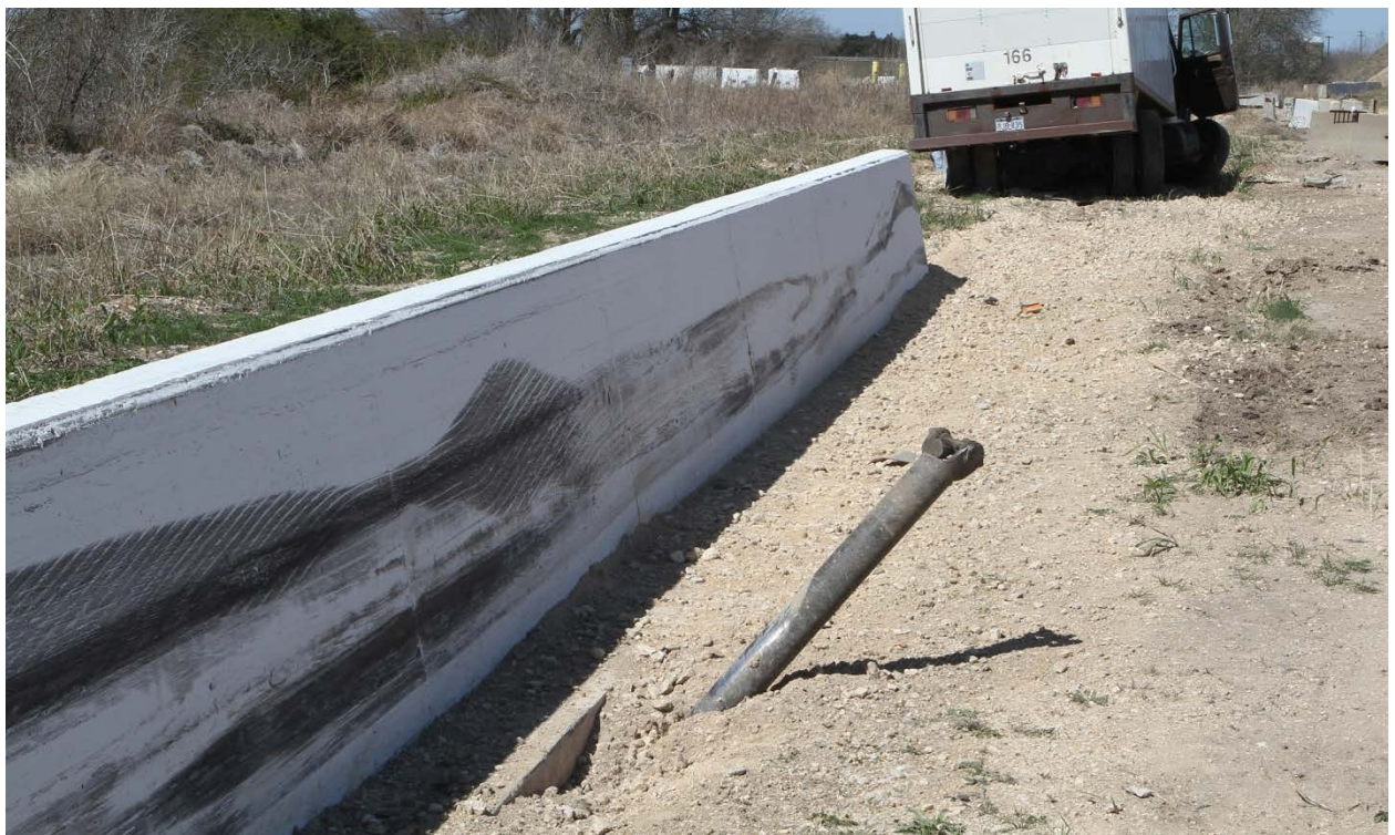
Figure 6.4. Installation After Test No. 420020-9b.
