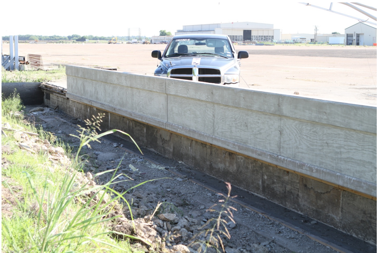
Figure 5.1. Vehicle/Installation Geometrics for Test No. 420020-3.
