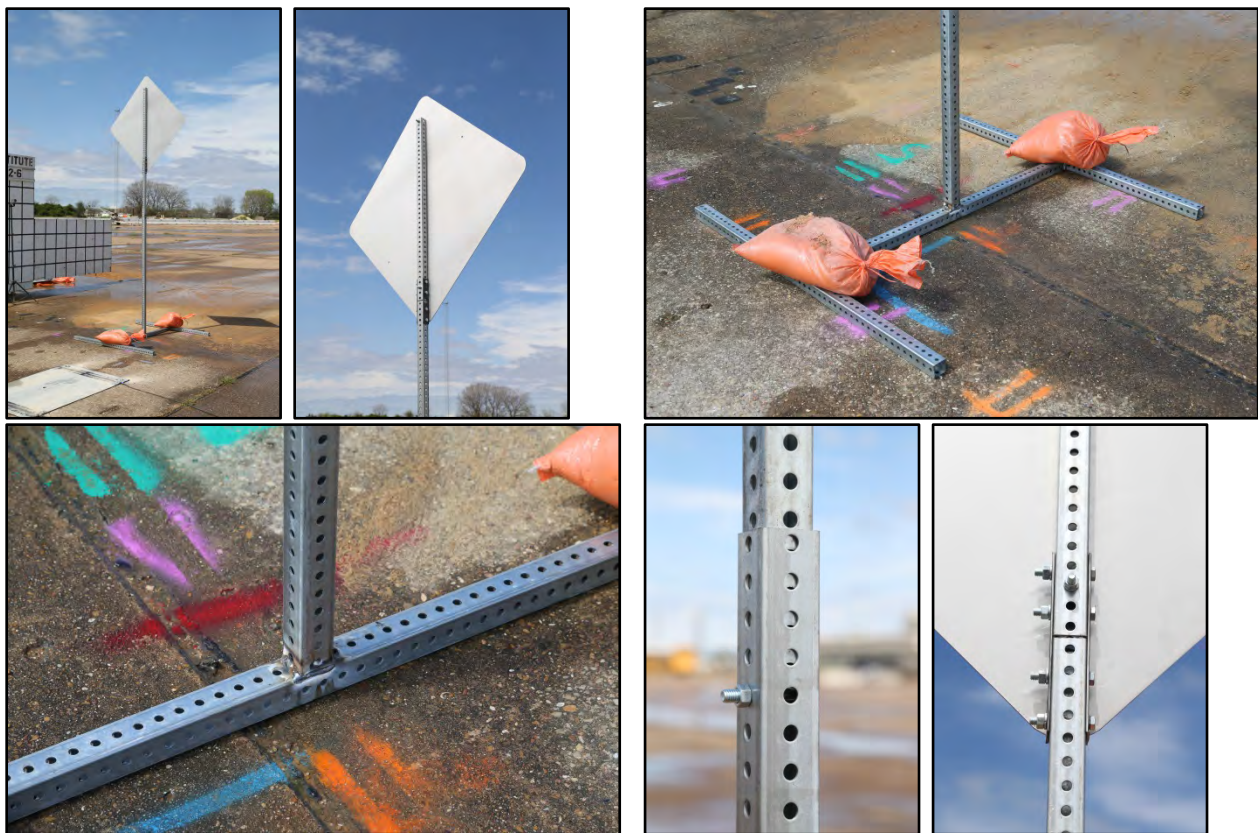
Figure 6.14. Option B Temporary Work Zone Sign Support Used for Test No. 490026-2-6.
