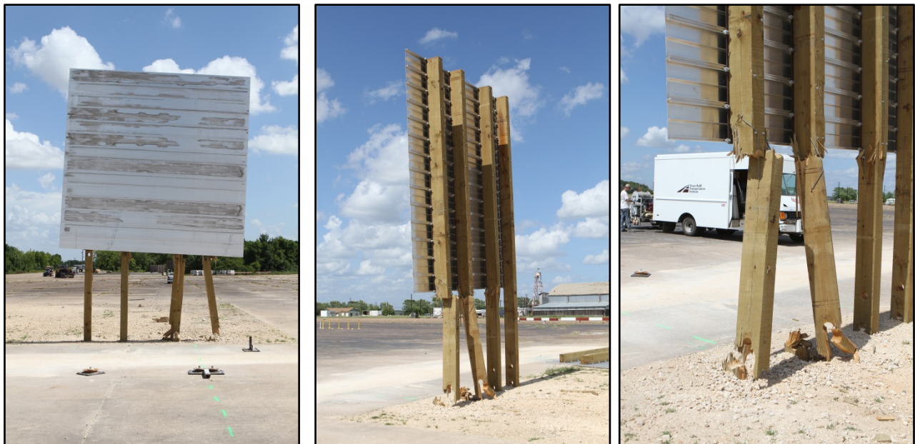
Figure 6.4. Installation after Test No. 490025-4-2.
