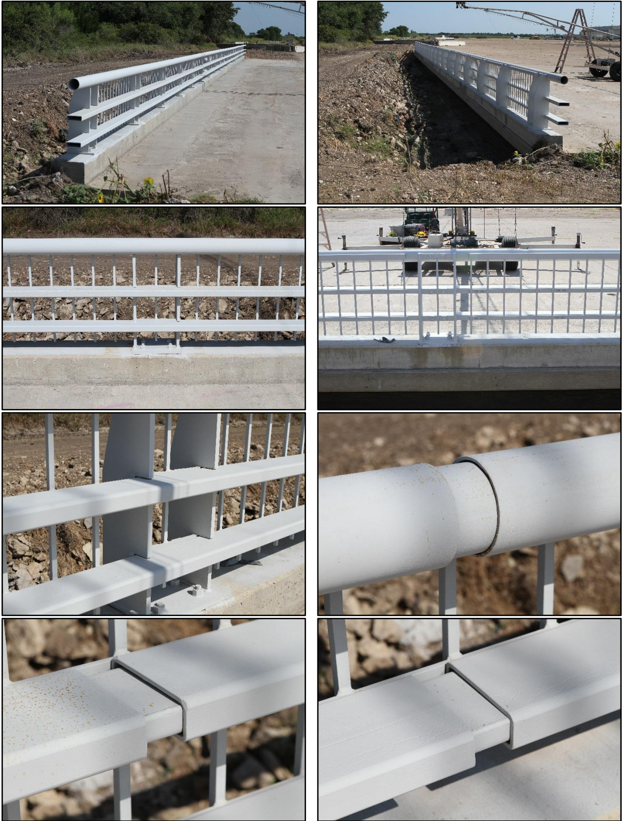
Figure 2-3. TxDOT Type C2P Bridge Rail prior to First Test 4-12.
