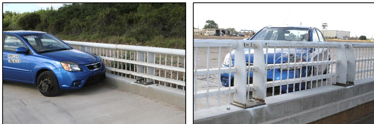
Figure 5-1. TxDOT Type C2P Bridge Rail/Test Vehicle Geometrics for Test No. 490026-4-1.
