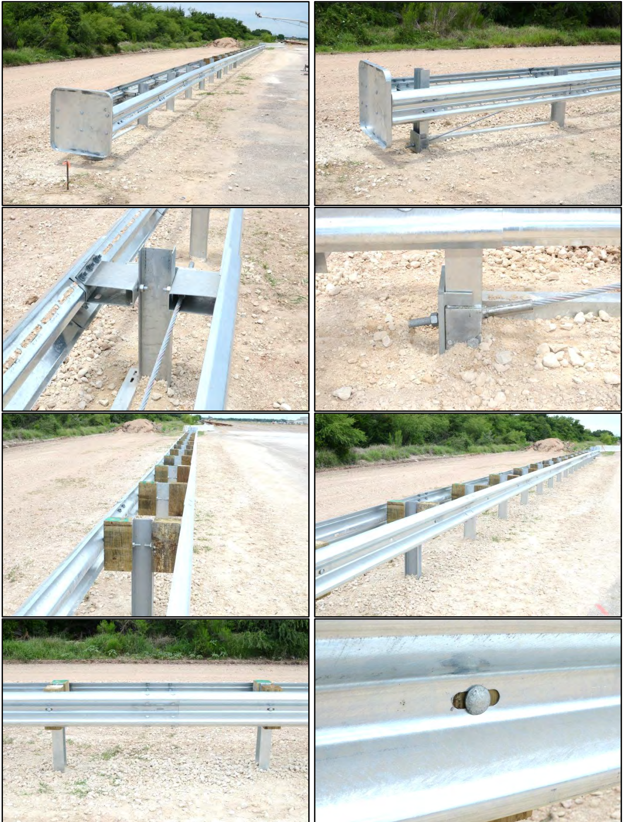
Figure 3.3. TxDOT 31-Inch W-Beam Median Barrier before Testing.
