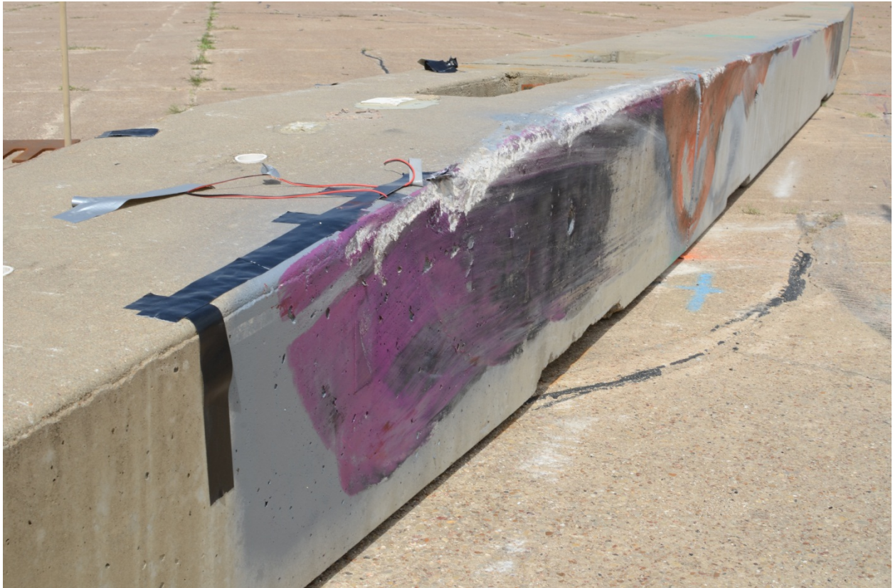
Figure 5.4. Installation after Test No. 490023-7.
