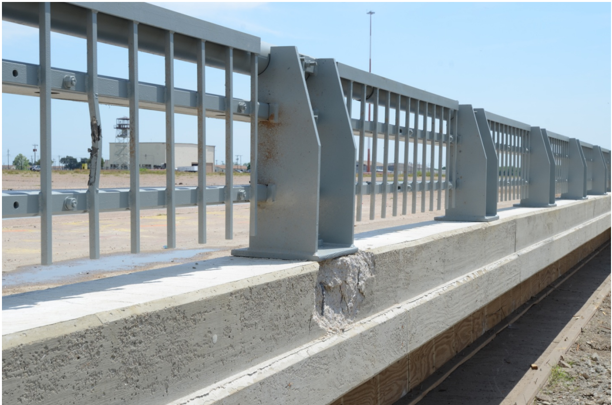
Figure 6.4. Installation after Test No. 490022-3.
