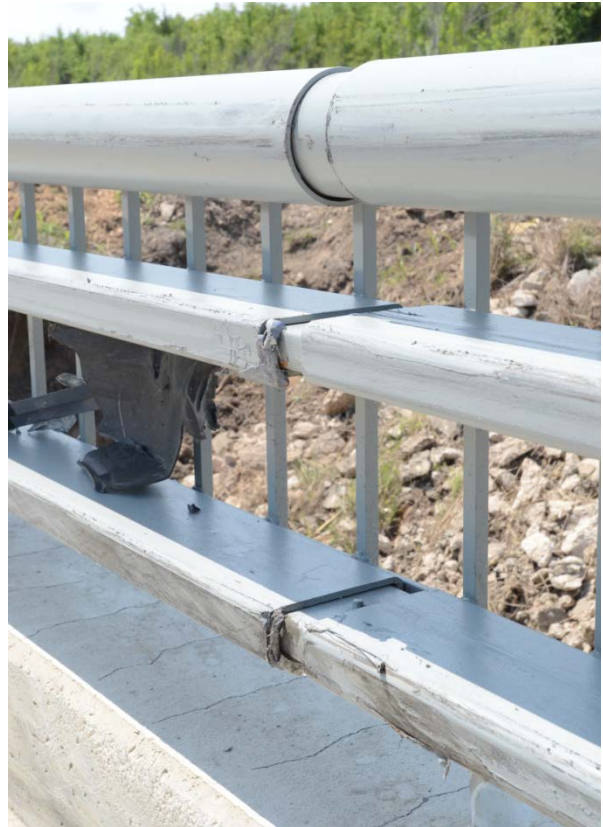
Figure 5.4. Installation after Test No. 490022-2.
