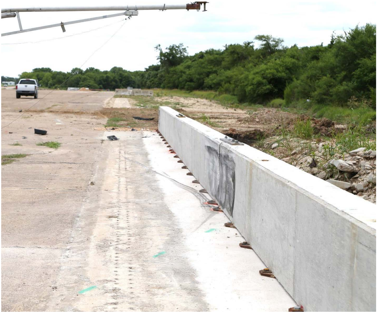
Figure 5.3. Vehicle/Bridge Rail after Test No. 490024-2-1.
