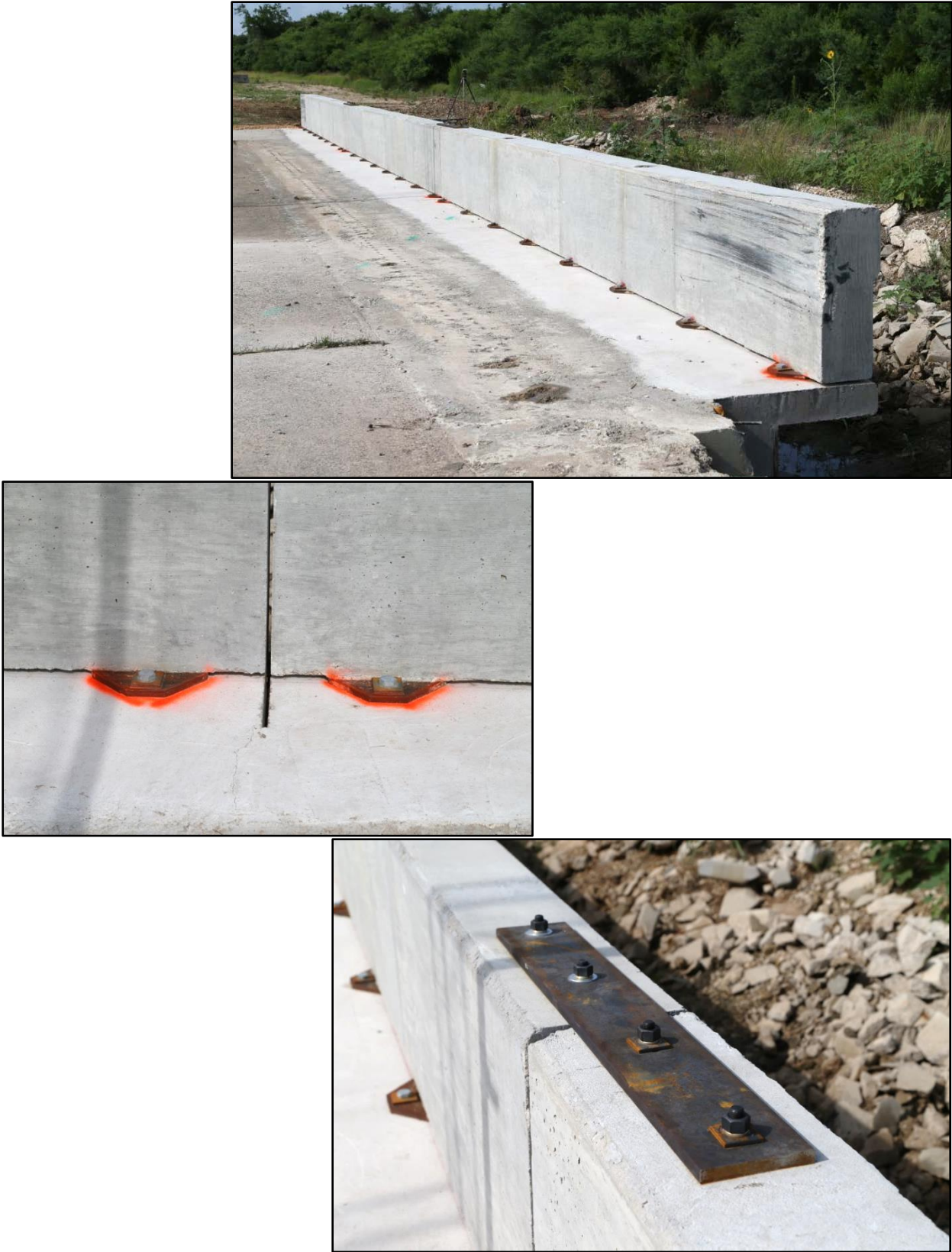
Figure 2.2. Test Article/Installation before Test No. 490024-2-1.
