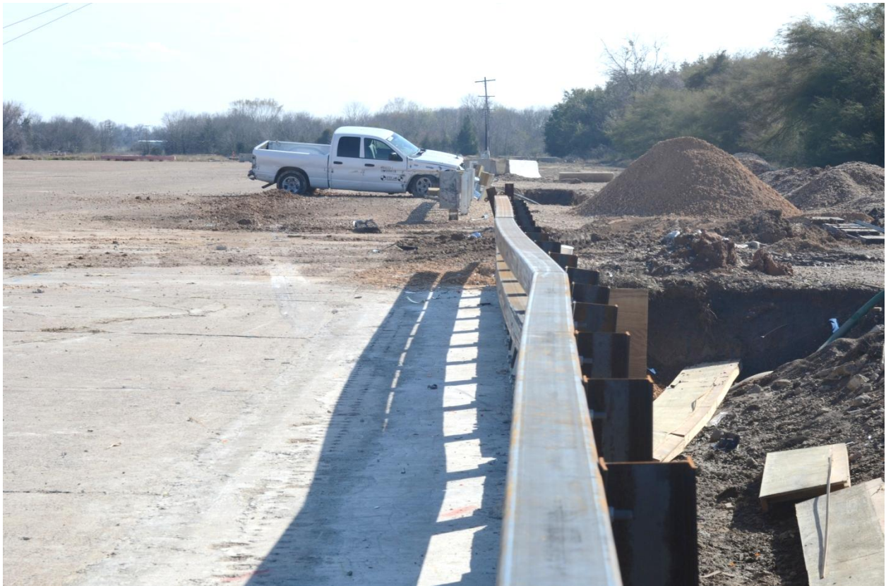
Figure 5.3. Vehicle/Installation after Test No. 490022-1.
