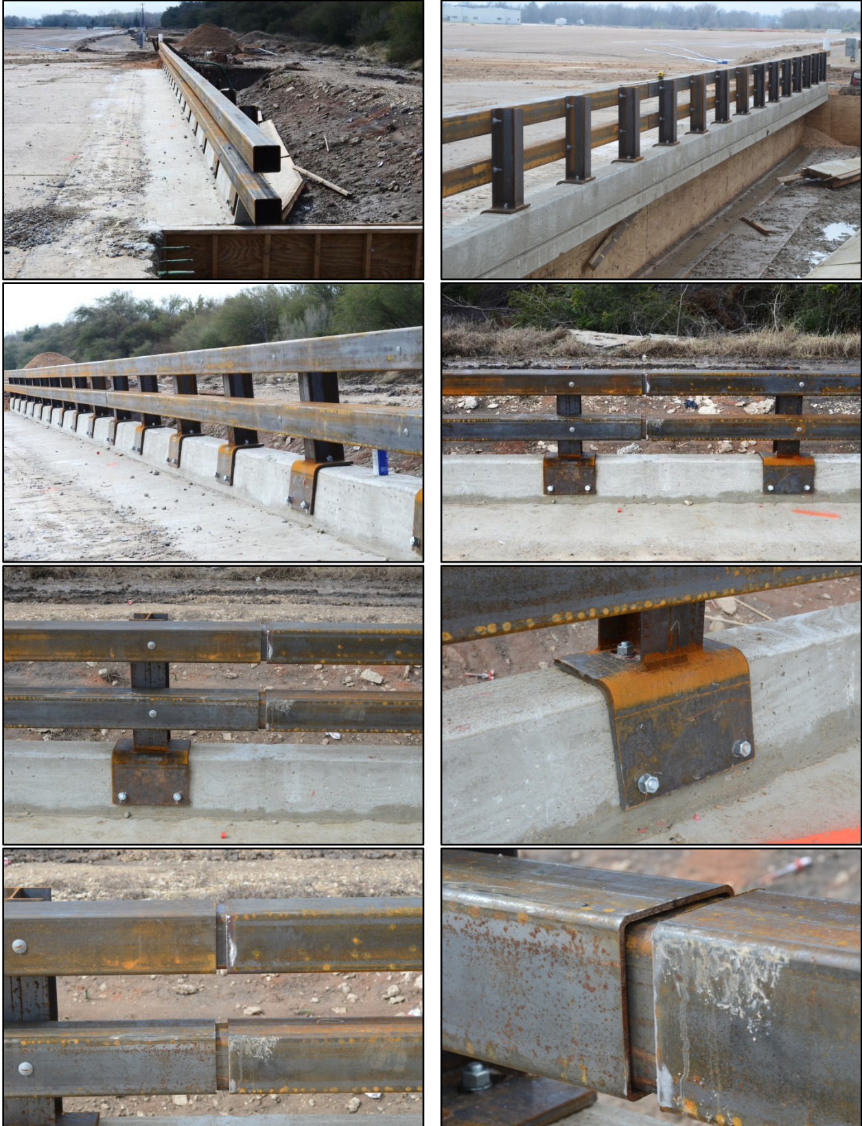
Figure 2.3. T131RC Bridge Rail Installation before Test No. 490022-1.
