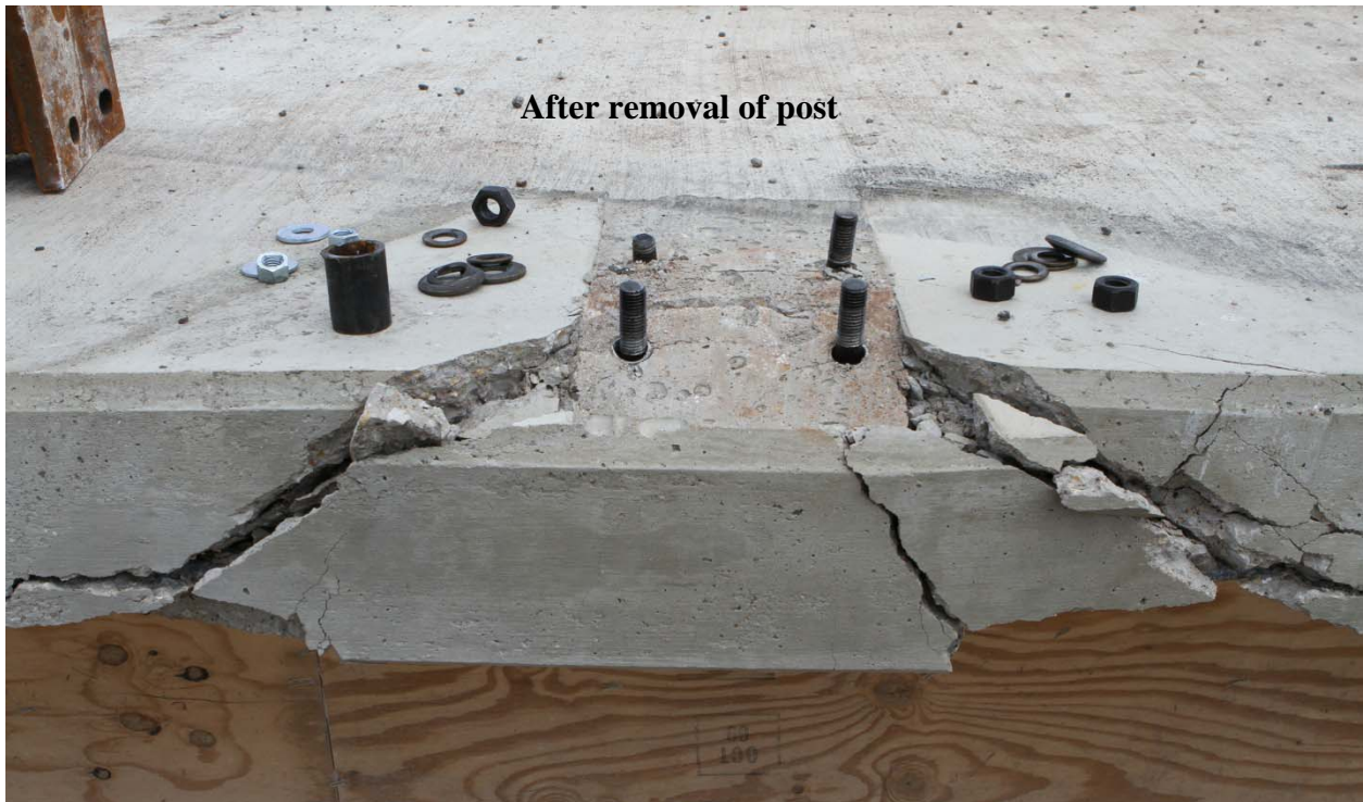
Figure 5.4. Installation after Test No. 420020-1a.
