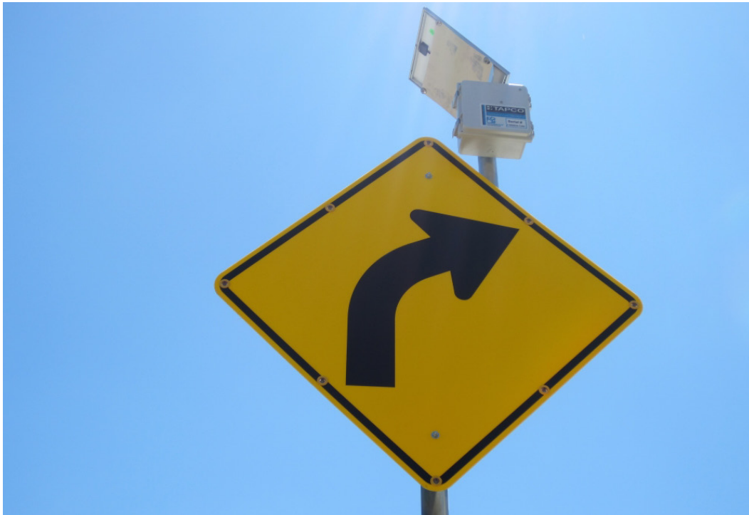
Figure 6. New Flashing Curve Warning Sign with Speed Activation and Solar Charging System.
