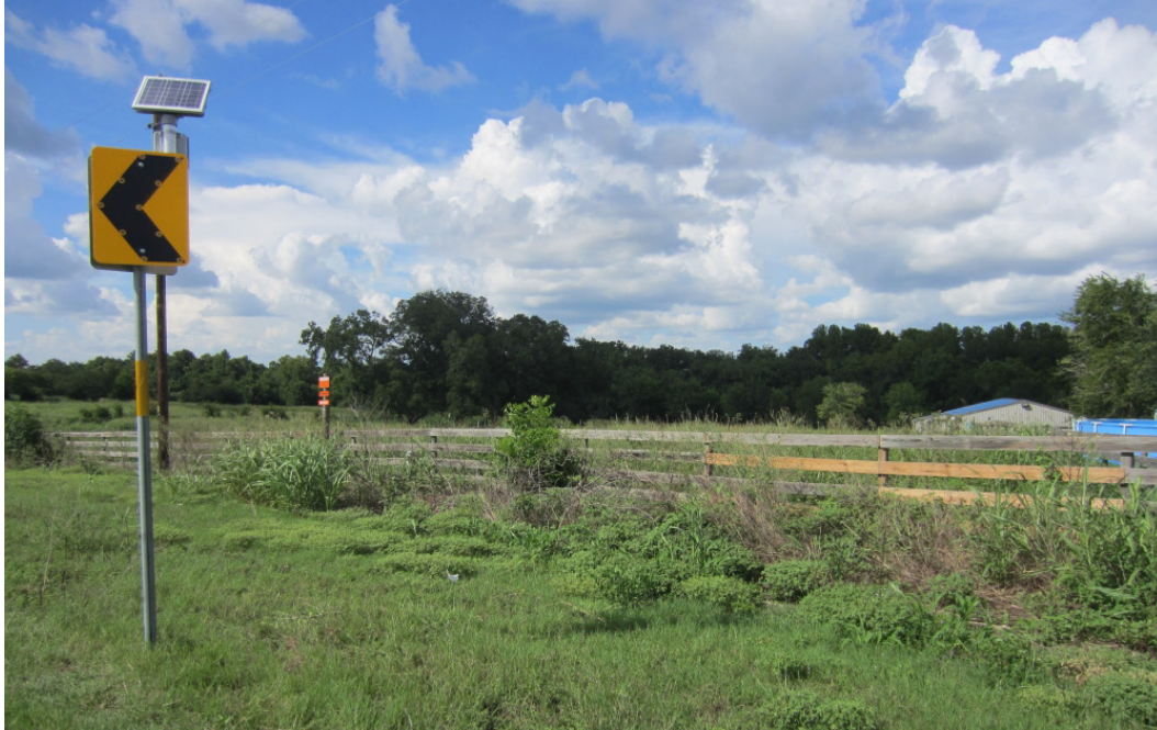
Figure 7. Installed Flashing Chevron near Where Vehicles Have Driven through Fence.
