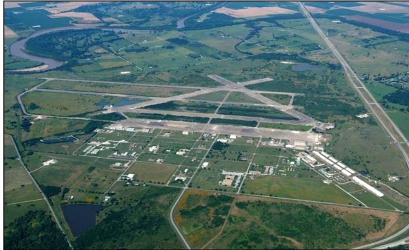
Figure 4. Riverside Campus Test Facility.
