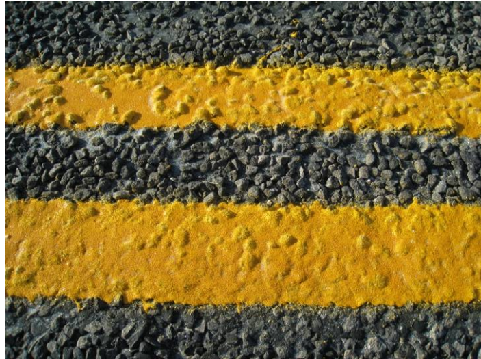
Figure 11. SH 85 Road Surface with Marking.
