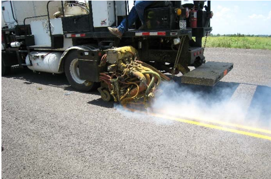
Figure 9. SH 21 Lead-Free Thermoplastic Installation.
