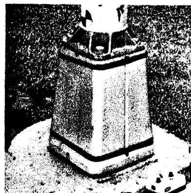
ALUMINUM POLE - ALUMINUM TRANSFORMER BASE
