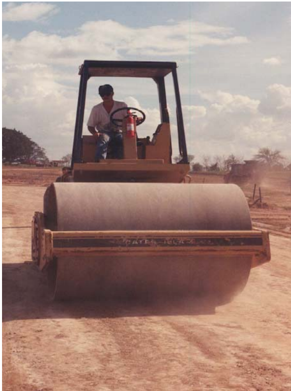
Figure 19. Pre-cracking Operations with Vibratory Roller (18).
