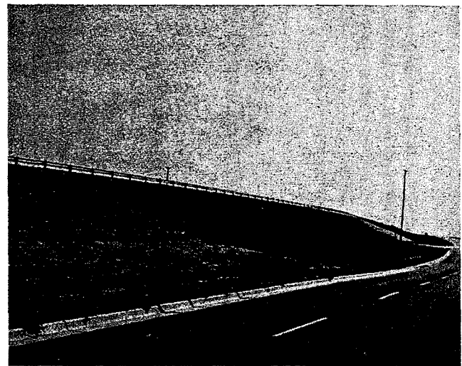
Figure 13. A surface mulch to conserve moisture in the seed zone is equally important in humid East Texas (top) as in the more arid climate of West Texas (bottom) to establish a permanent plant cover. Unmulched areas seeded with perennial grasses supported only a thin cover of annual plants which soon disappeared with the onset of hot dry weather and left the slopes subject to erosion.
