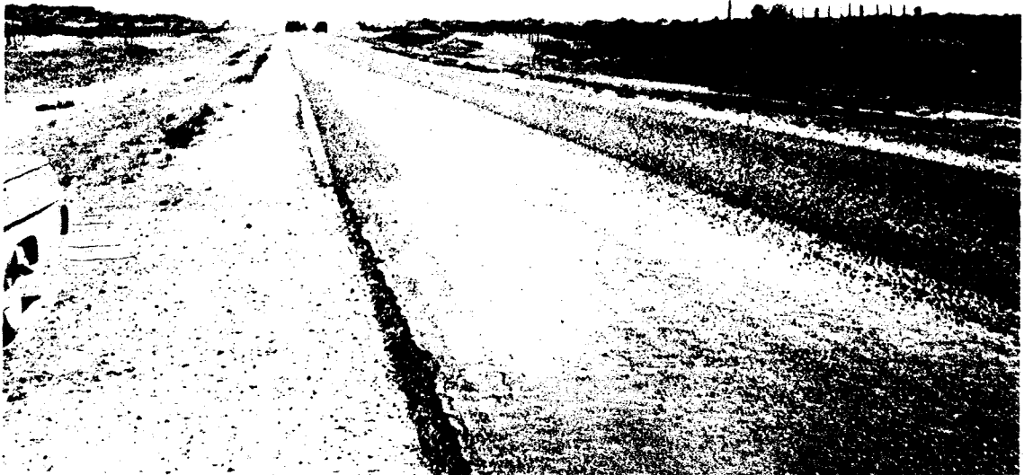
FIGURE 52 Patches create variations in asphalt demand of surface.
