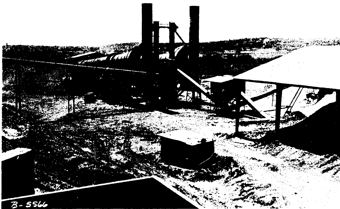
Figure 3. Shale storage and conveyor feed to kilns. (Photo by Gustafson.)
