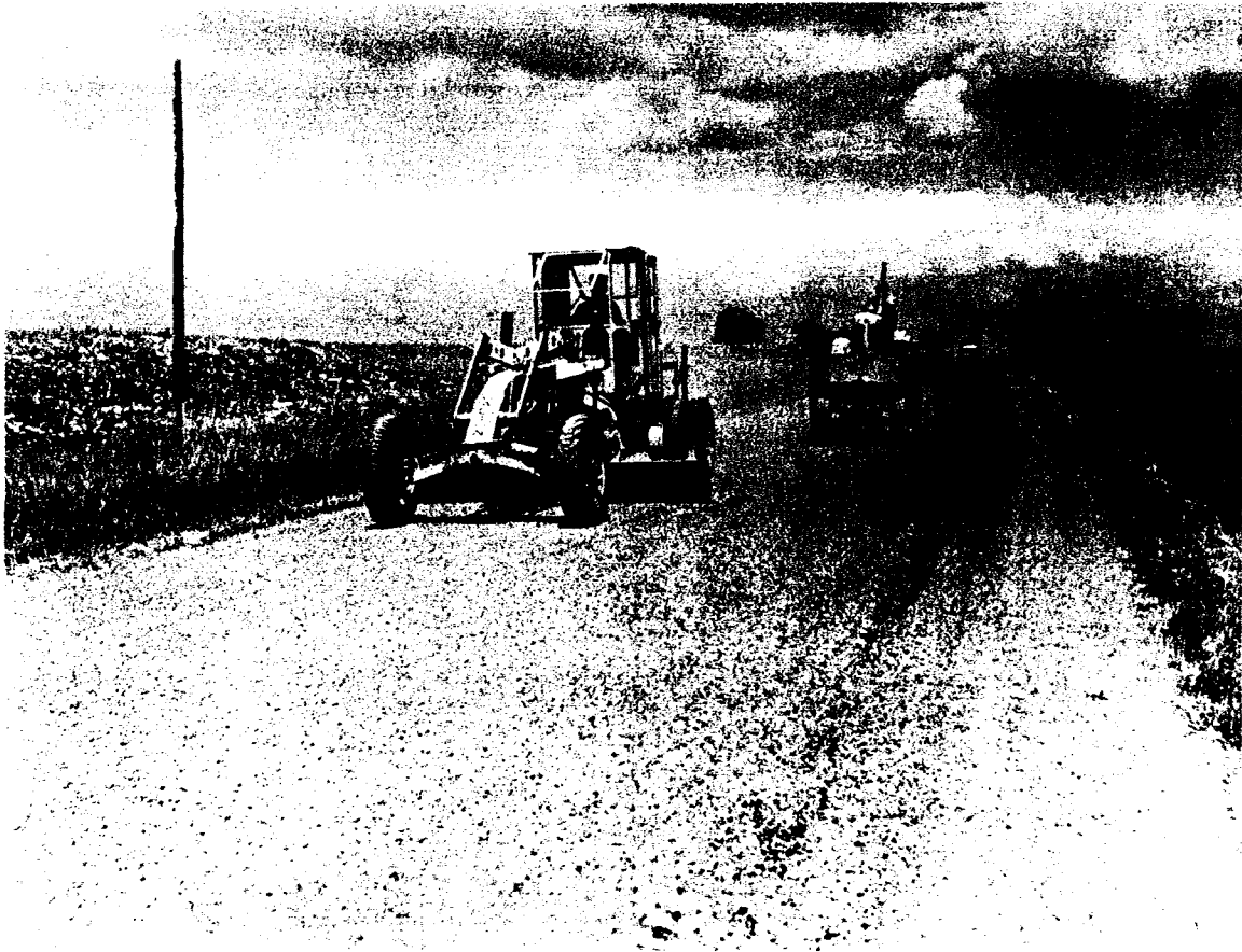
FIGURE 61 Blade broom successfully used on Type F coverstone. (Photo by Gustafson.)
