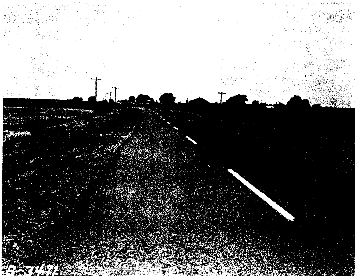
FIGURE 58 Typical farm-to-market road surfaced with Type F material. (Photo by Gustafson.)
