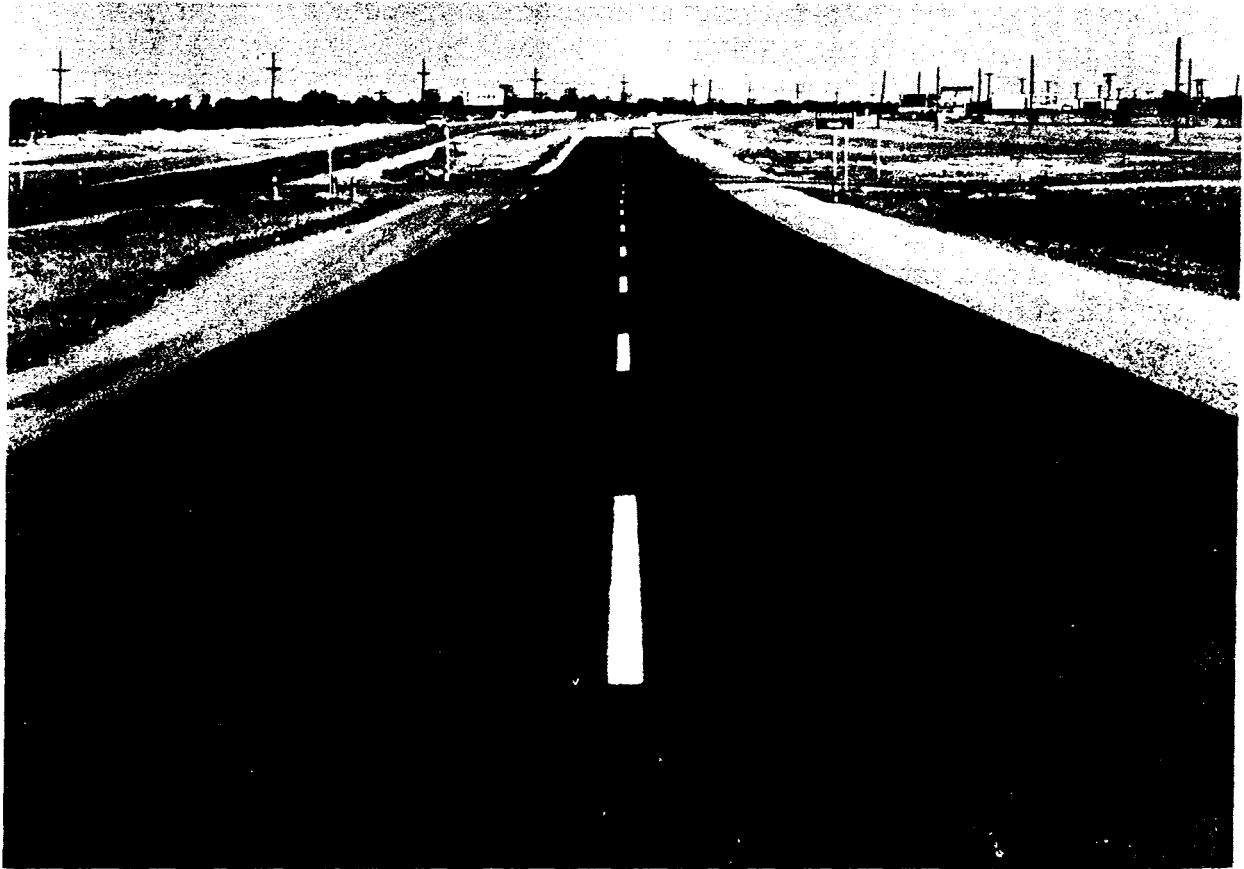
FIGURE 48 Type F seal two years old with 7700 vpd. (Photo by Billingsley and Plumlee.)
