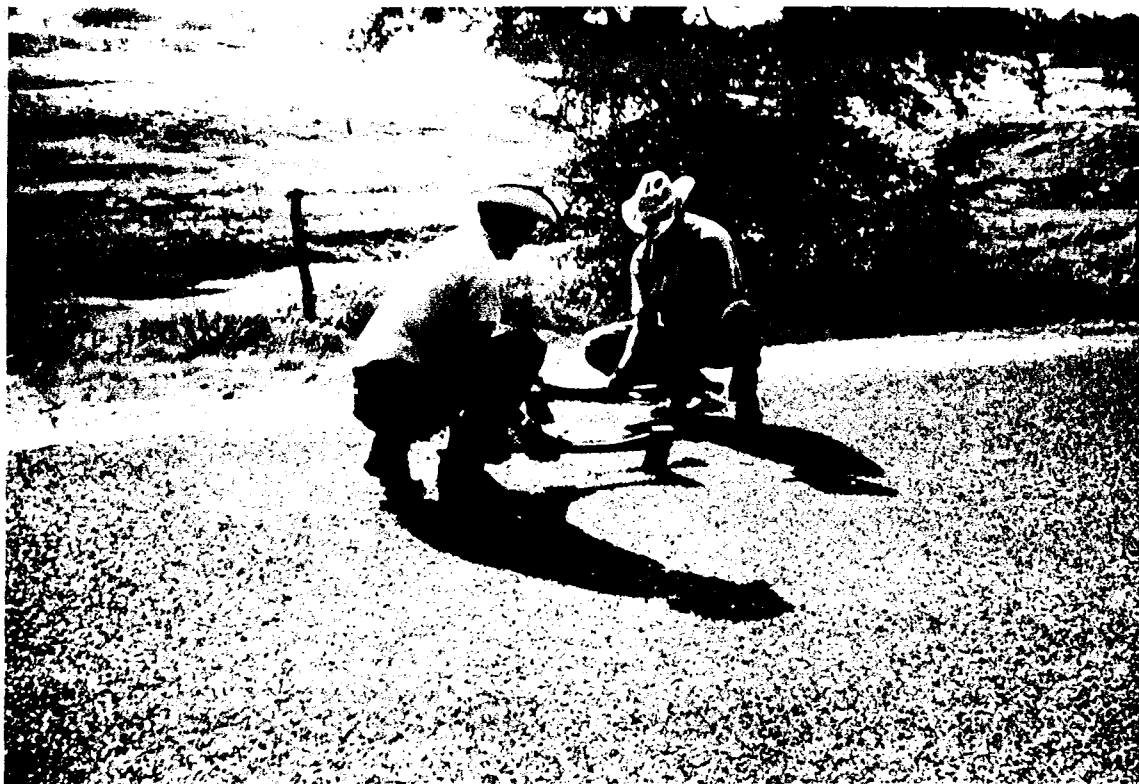
FIGURE 41 Cutting a field sample with an ax.
