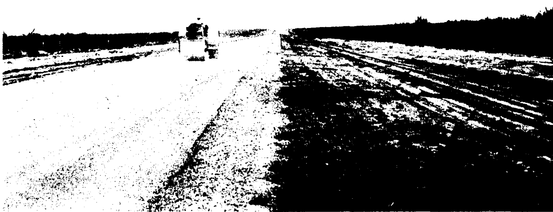
FIGURE 53 Experimental section proves that the use of steel flat wheel roller is not advisable.
