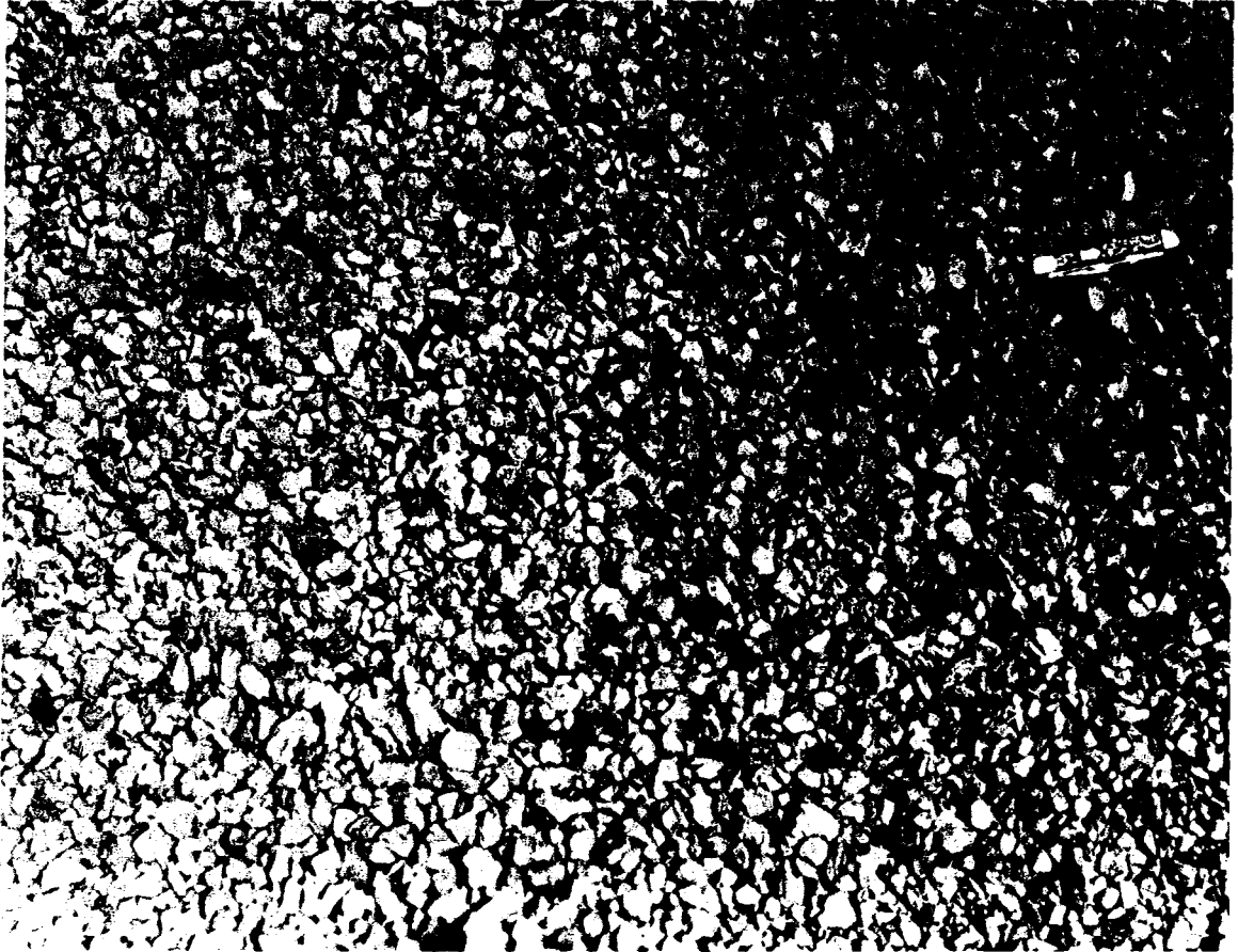
FIGURE 63 Type F Grade 3 after brooming. Spread rate -- 130 square yards per cubic yard. (Photo by Gustafson.)
