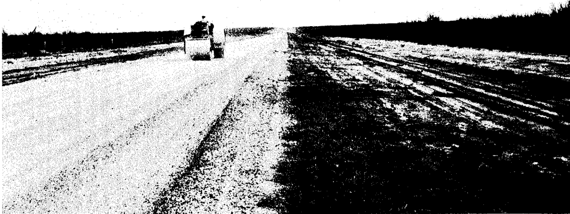
Figure 49. Experimental section proves that the use of steel flat wheel roller is not advisable.
