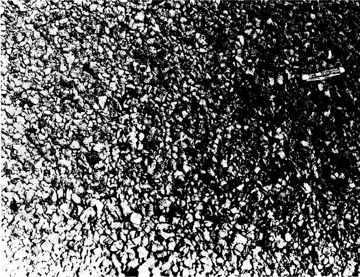
Figure 59. Type F Grade 3 after brooming. Spread rate -- 130 square yards per cubic yard. (Photo by Gustafson.)
