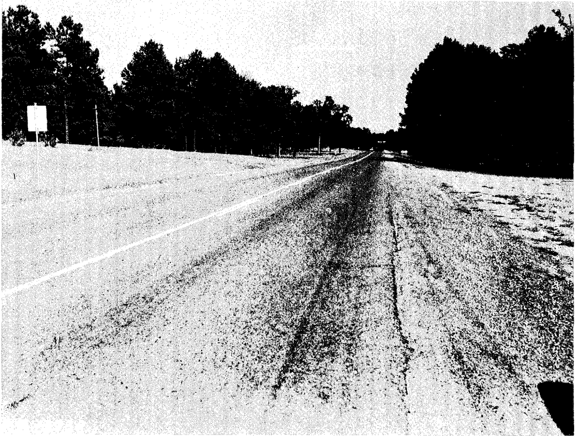
Figure 56. Type F cover aggregate in service three months, 1500 vpd, U S 190. (Photo by Gustafson.)
