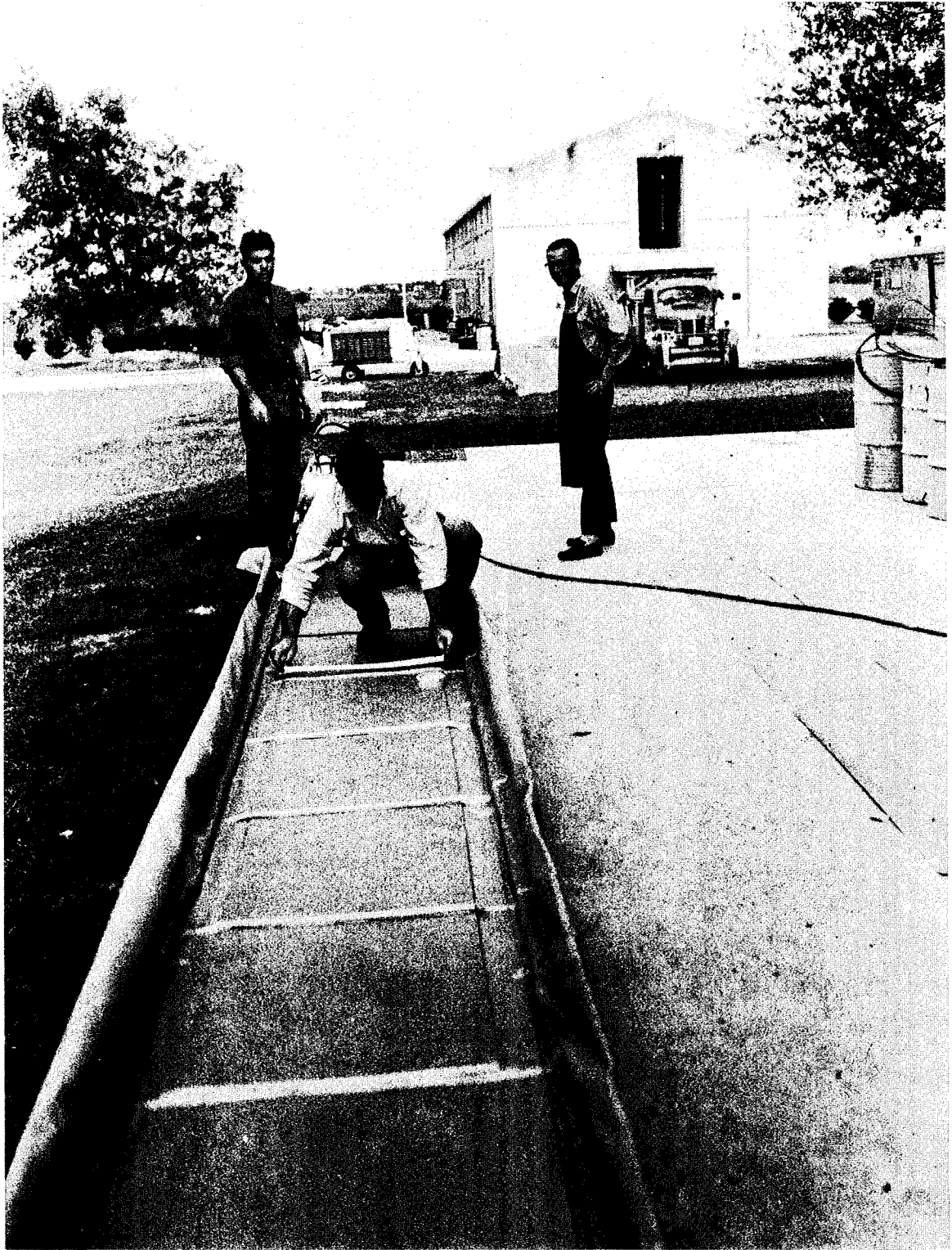
Figure 10. Boards in line for asphalt shot.
