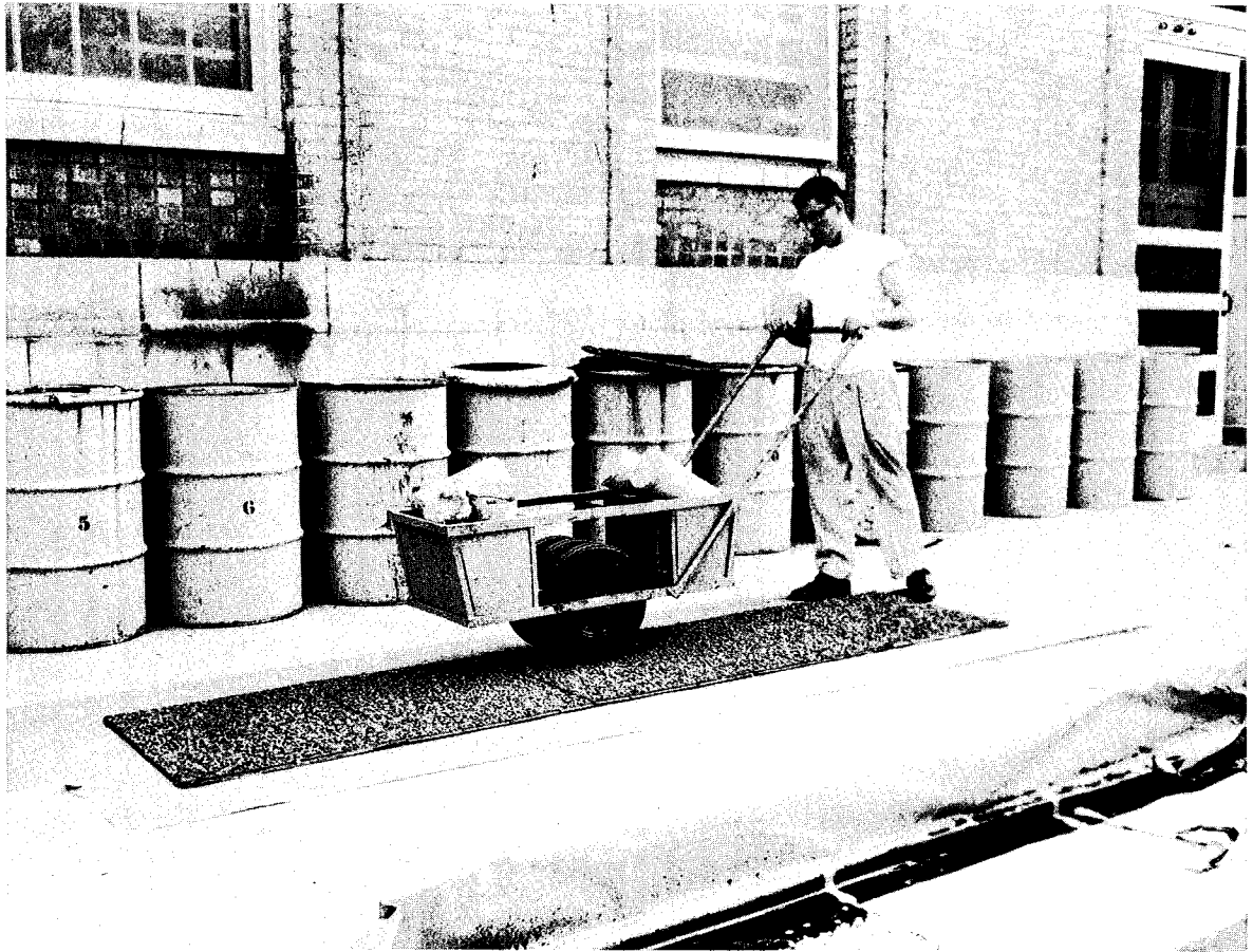
Figure 15. Pneumatic roller used to seat stone on laboratory surface treatments.
