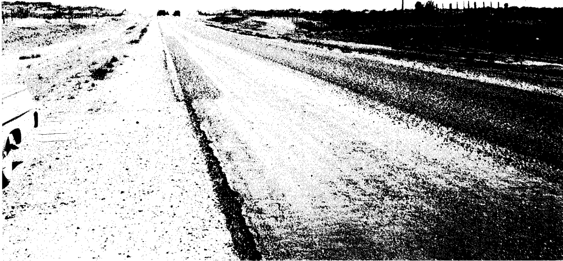
Figure 48. Patches create variations in asphalt demand of surface.
