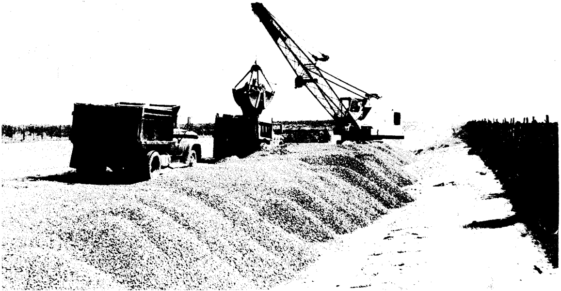
Figure 46. Stockpile and loading operation of Type F material.
