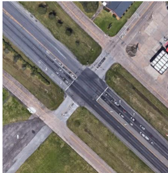
Figure 48. Intersection of US 60 and 30th Street.
