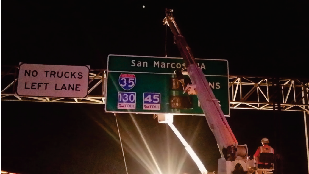
Figure 1. Travel Time Sign Being Installed at Site 1.
