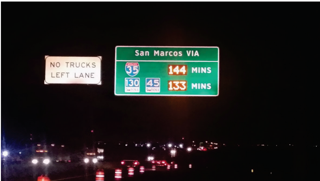
Figure 2. Installed Sign at Site 1 Illustrating Successful Testing of the DMS Insets.
