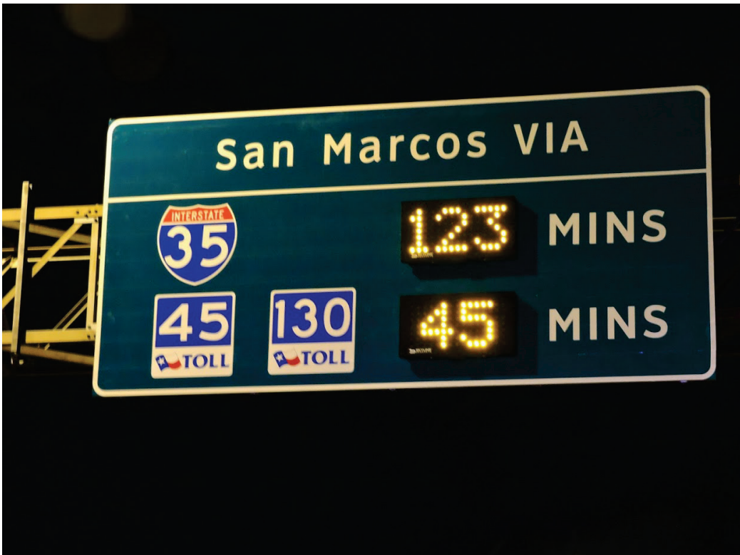
Figure 5. Installed Sign at Site 2 Illustrating Successful Testing of the DMS Insets.
