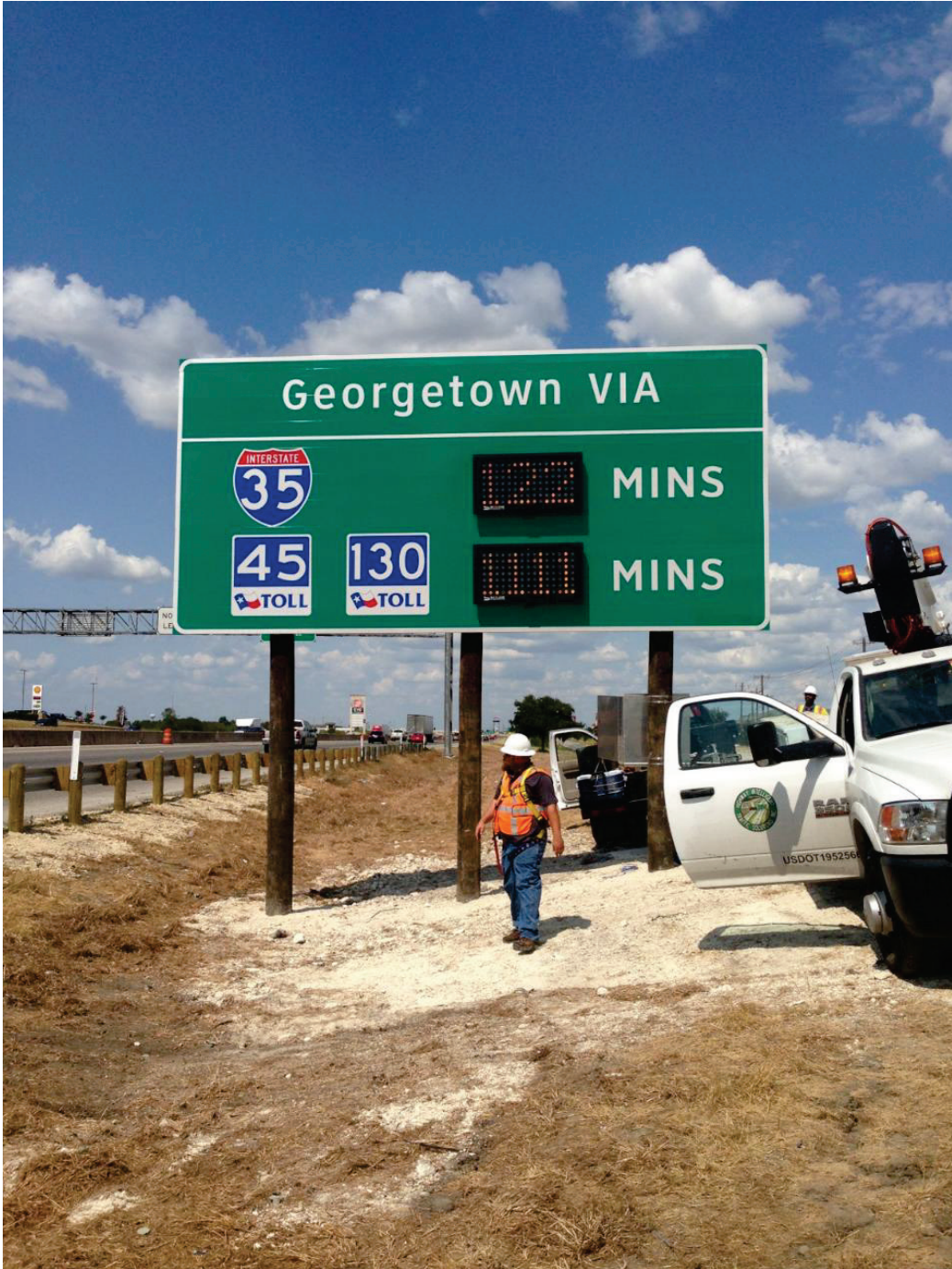
Figure 8. Installed Sign at Site 3 Illustrating Successful Testing of the DMS Insets.
