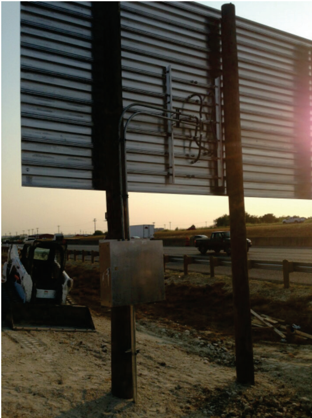
Figure 7. Travel Time Sign Being Installed at Site 3.
