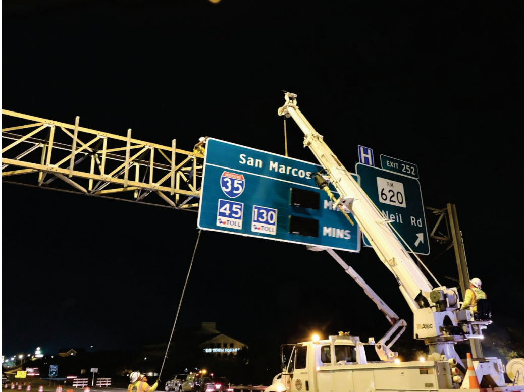
Figure 4. Travel Time Sign Being Installed at Site 2.
