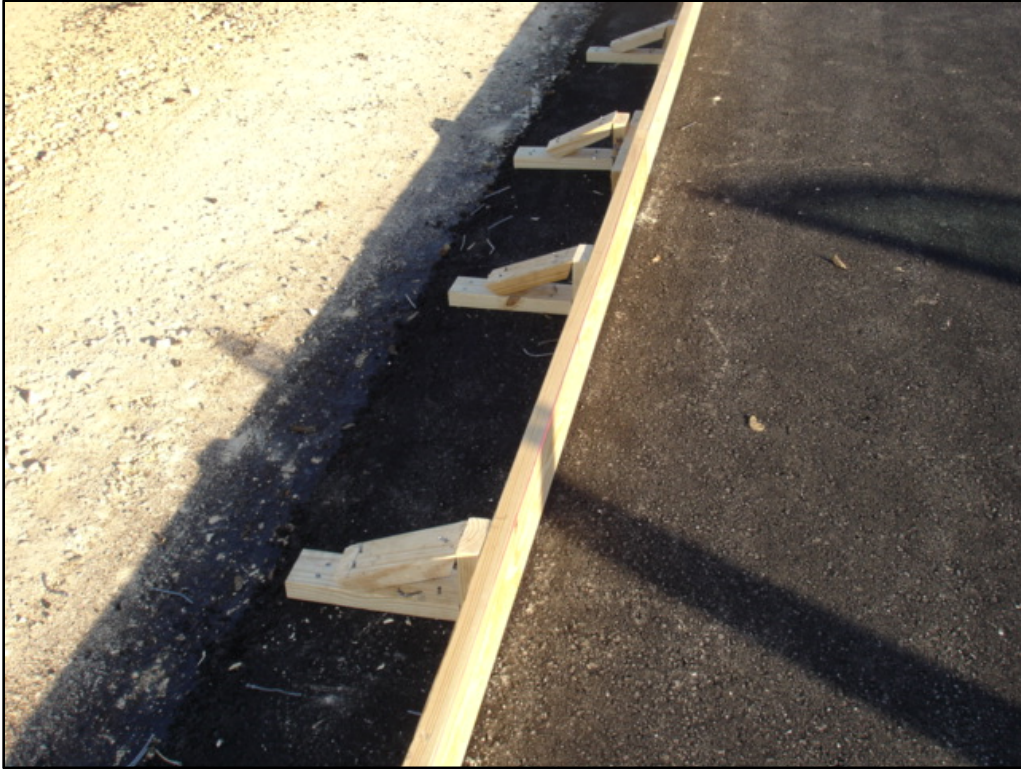
Figure 33. Form along West Side of Type C Base to Place CRCP.
