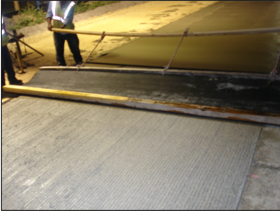
Figure 38. Concrete Surface Textured with Carpet Drag.
