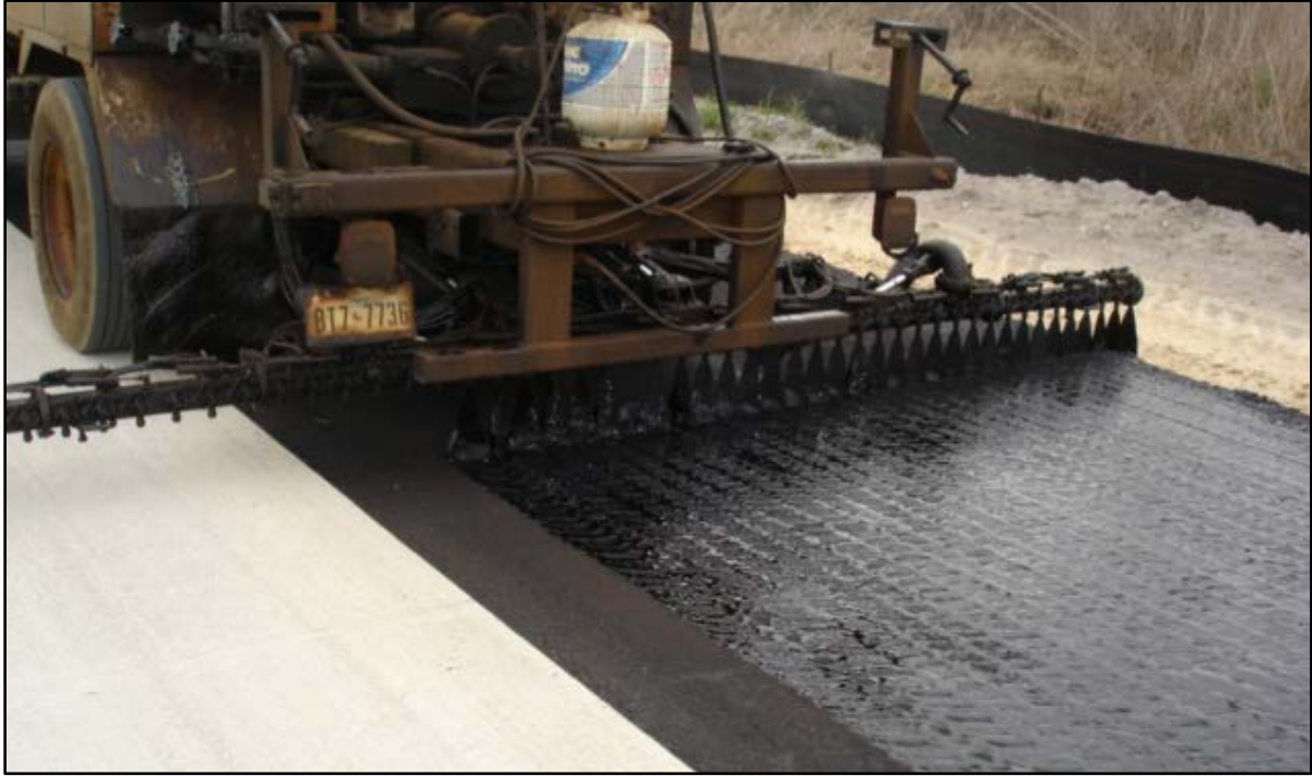
Figure 44. Asphalt Sprayed on Flexible Base for Surface Treatment.
