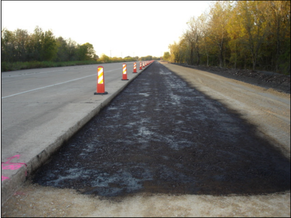
Figure 30. Tack Coat Applied to Flexible Base.
