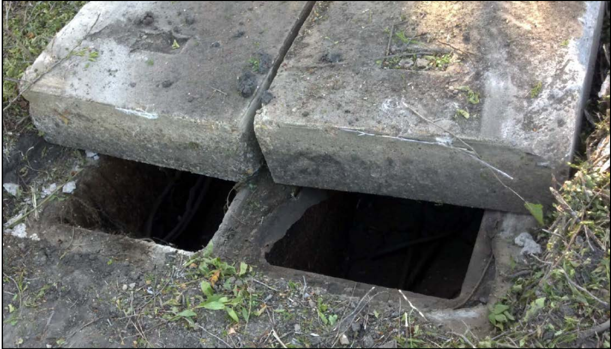
Figure 23. Utility Box Found within Construction Site.
