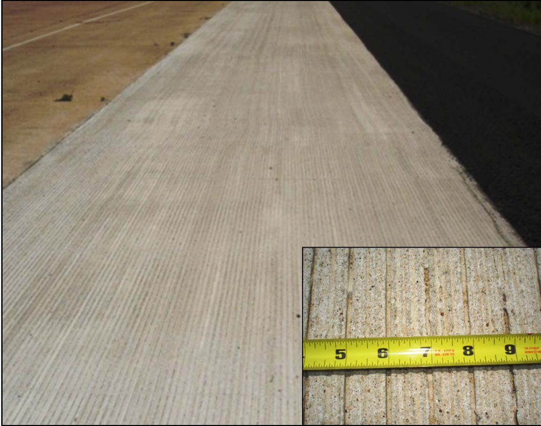
Figure 51. One-inch Longitudinally Tined CRCP Section.
