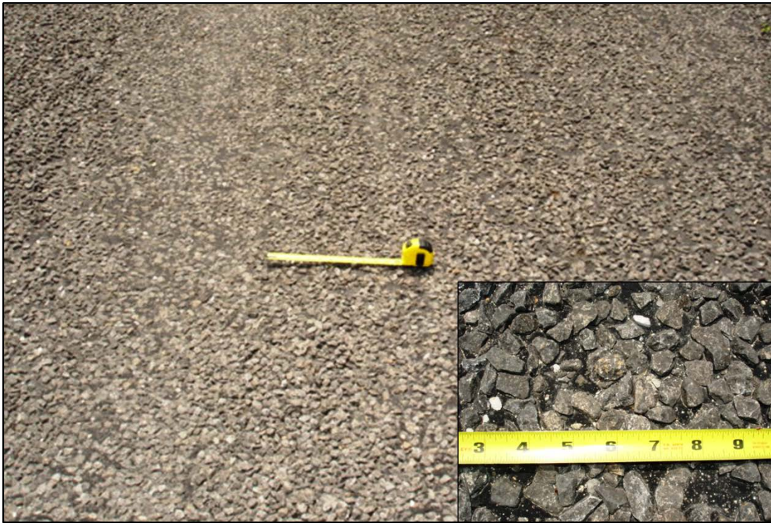
Figure 56. Grade 3 Chip Seal Section.
