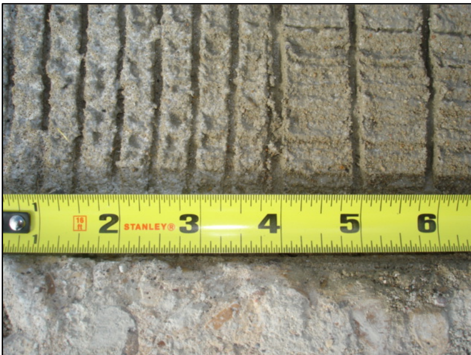
Figure 41. Change from 1/2-inch to 1-inch Transverse Tines.
