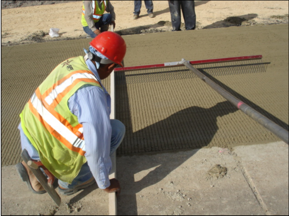
Figure 42. Concrete Surface Texture with 1-inch Transverse Tines.
