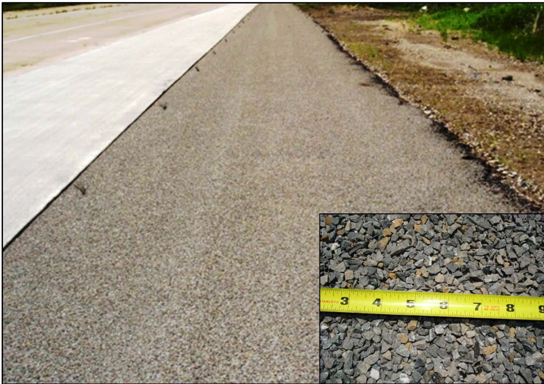
Figure 55. Inverted Prime Section.
