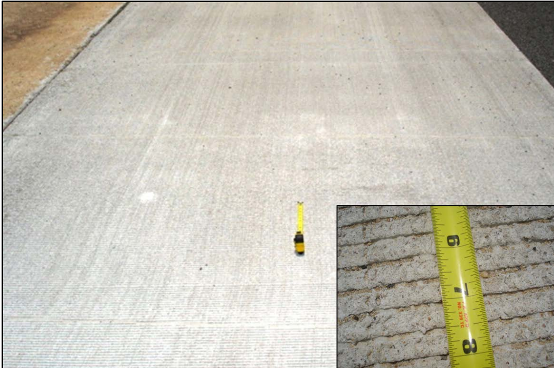
Figure 52. Half-inch Transversely Tined CRCP Section.
